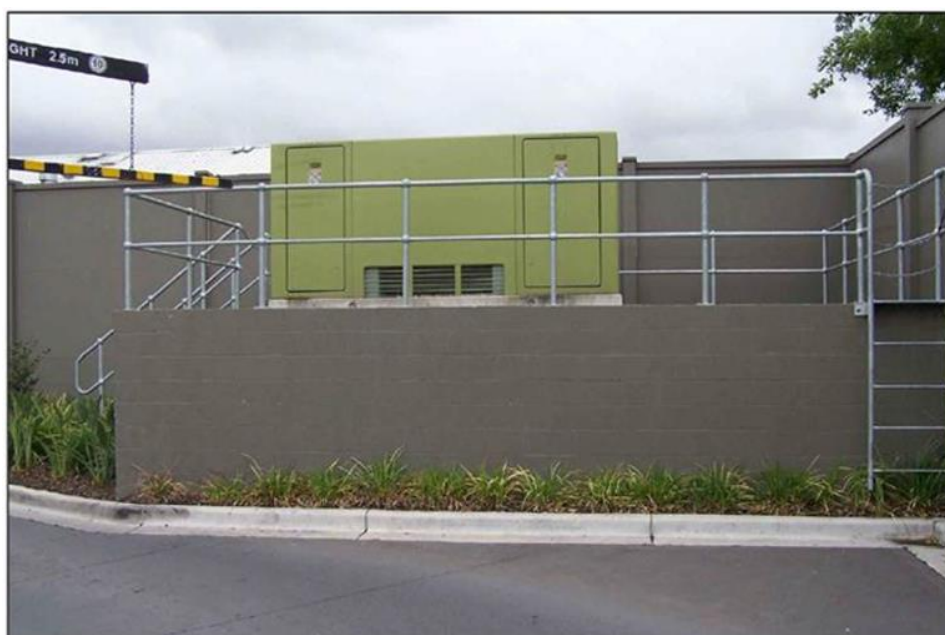
Figure 51 - Example substation raised above 1:100 flood level
