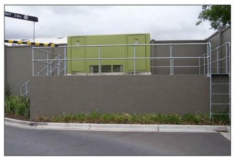
Figure 51 - Example substation raised above 1:100 flood level
