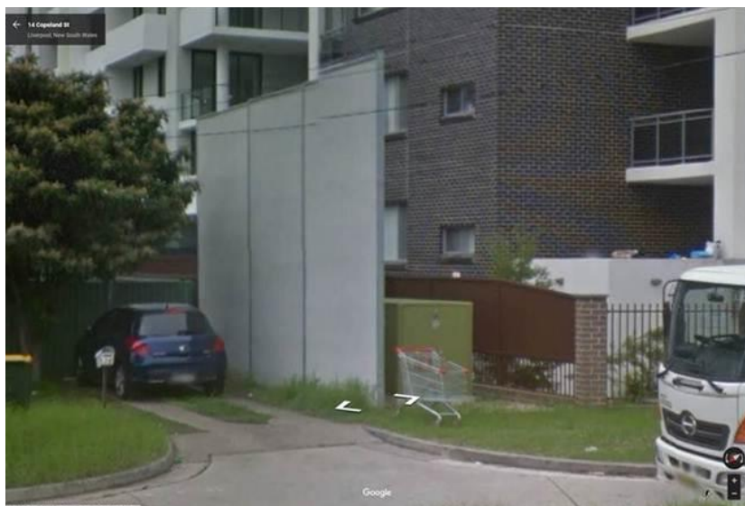
Fire wall constructed for padmount substation in Liverpool. Source: Google Maps Street View.
