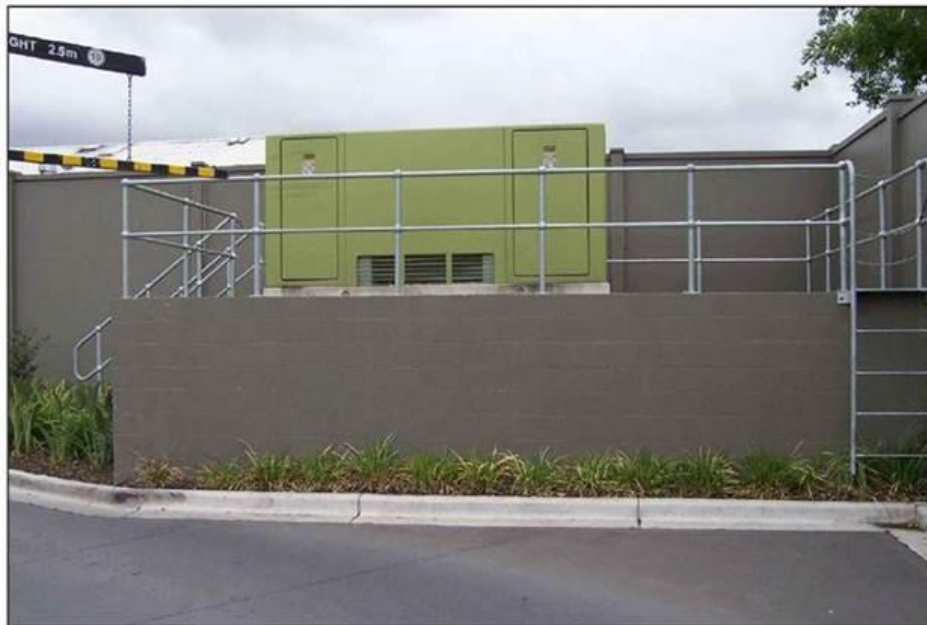
Figure 51 - Example substation raised above 1:100 flood level
