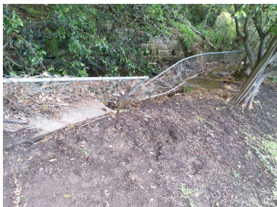
Following 29 Nov 2018 sheet flooding of Oval, Chain-wire fence shows debris-tide line about 300mm high, and fence and stone retaining wall are washed into creek by force of direction of water escape flow.
