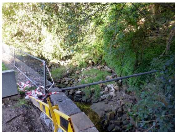
March 2019, storm-eroded rocks lie in creek bed; stone creek wall and playground edge still need repair.
