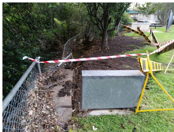
Following 29 Nov 2018 sheet flooding of Oval, Chain-wire fence shows debris-tide line about 300mm high, and fence and stone retaining wall are washed into creek by force of direction of water escape flow.
