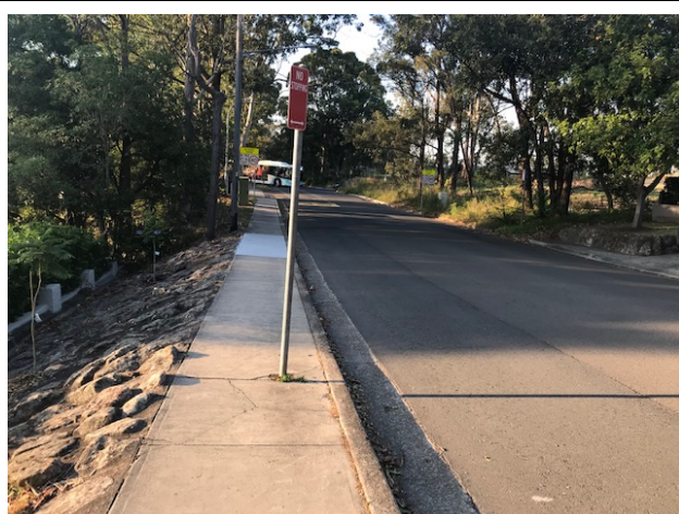
Photo 11 - Footpath north of bus stop too narrow, sign obstructs path, no runoff, path expected to be shared by pedestrians & cyclists
