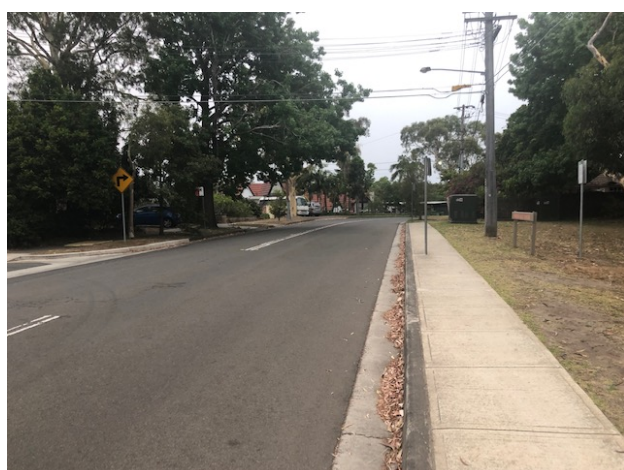
Photo 15 - Eton Road footpath not continuous, and against the kerb. Pedestrians are forced to cross the road at the corner without good visibility (this section has a bus stop and vehicles are forced around the bus). refer also Photo 6
