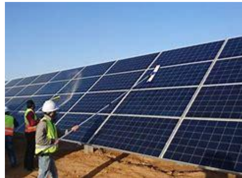
Cleaning PV solar panels
