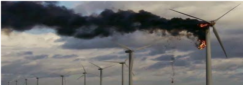
Wind turbine on fire
