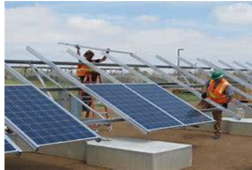
Crew of two install cross-members and panels
