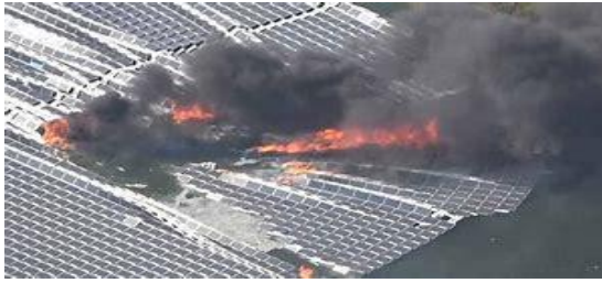
PV solar IEGW left to burn out
