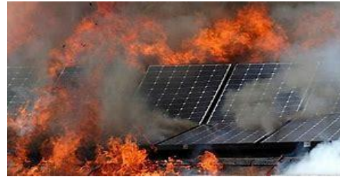
PV solar panel fire
