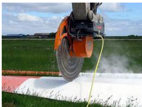
Cutting up end-of-life wind turbine blades
