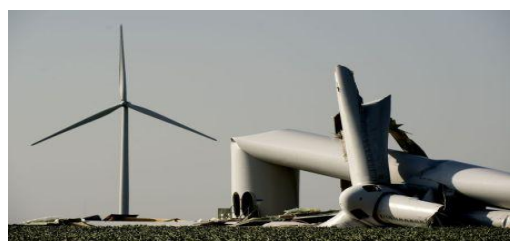
Wind turbine collapse
