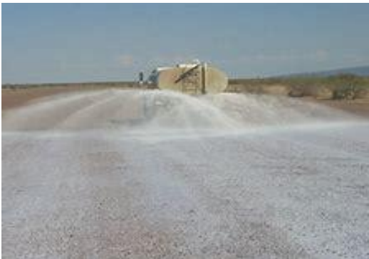
Construction site dust control
