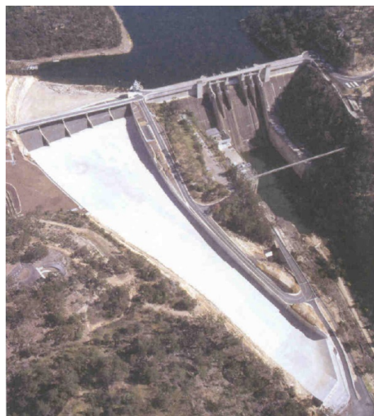
Figure 3.12: Overhead view of the newly completed auxiliary spillway, 2002 (Source: SCA)
