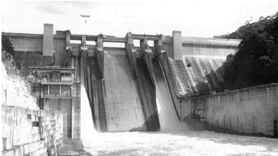
Figure 3.10: Photograph showing the raising of the crest wall using the 18 tonne cableway that remained at this time, November 1988. (Source: R95B – 2, SWC/SCAHR&AF)
