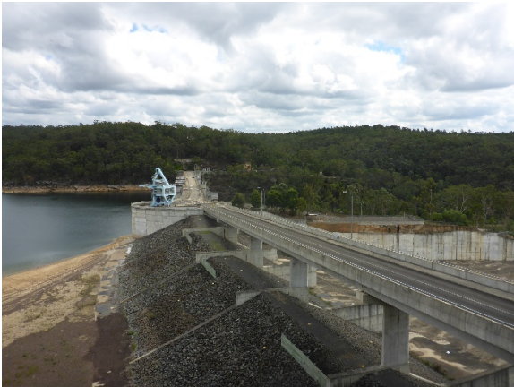
Figure 4.14: View north-west to existing bridge on Production Avenue over auxiliary spillway and crest road on the dam wall, note blue crest crane in distance.
