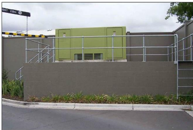
Figure 51 - Example substation raised above 1:100 flood level
