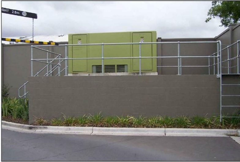
Figure 51 - Example substation raised above 1:100 flood level
