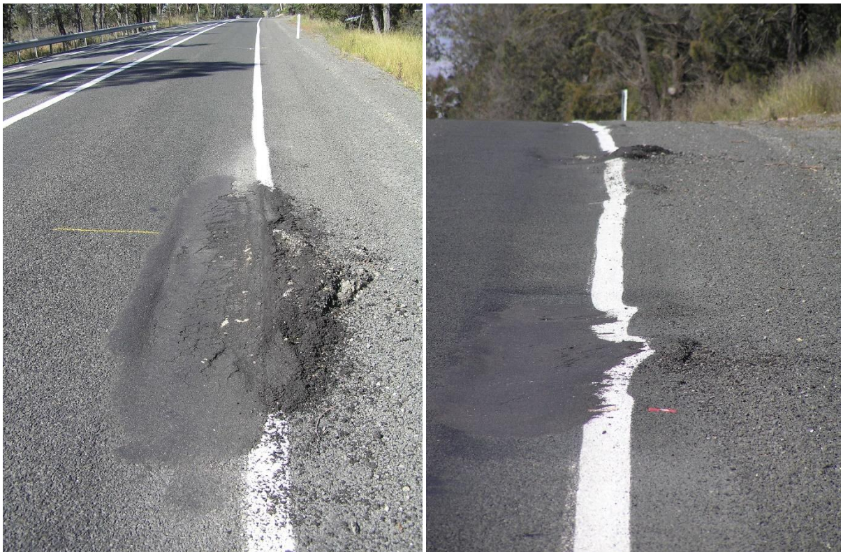
Brayton Road_Photos #16 and #17_Damaged sections after patching_18Apr21
