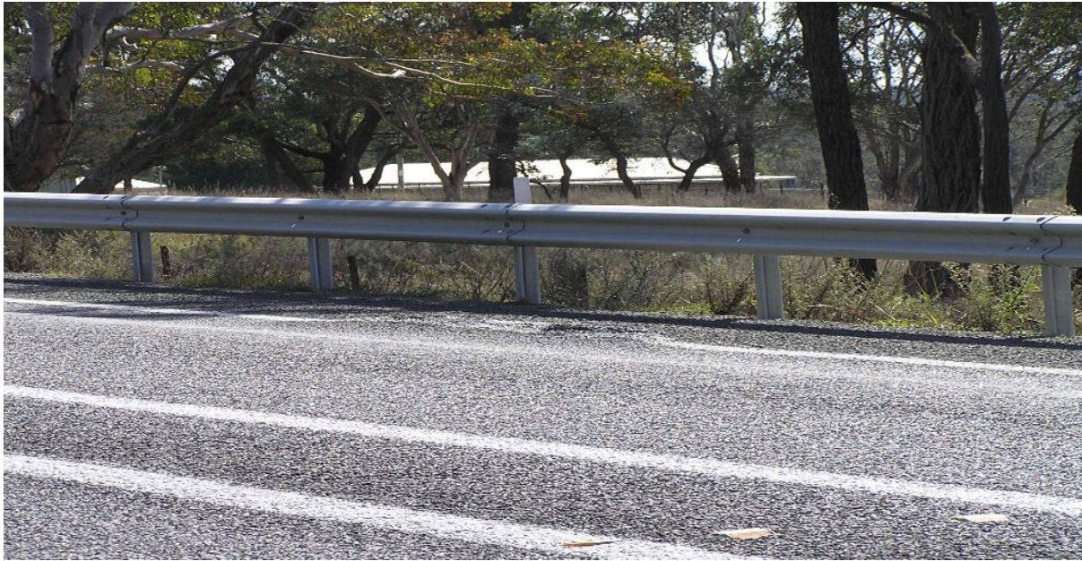
Brayton Road_Photo #15_ deep rut close to guard rail. _18Apr2021
