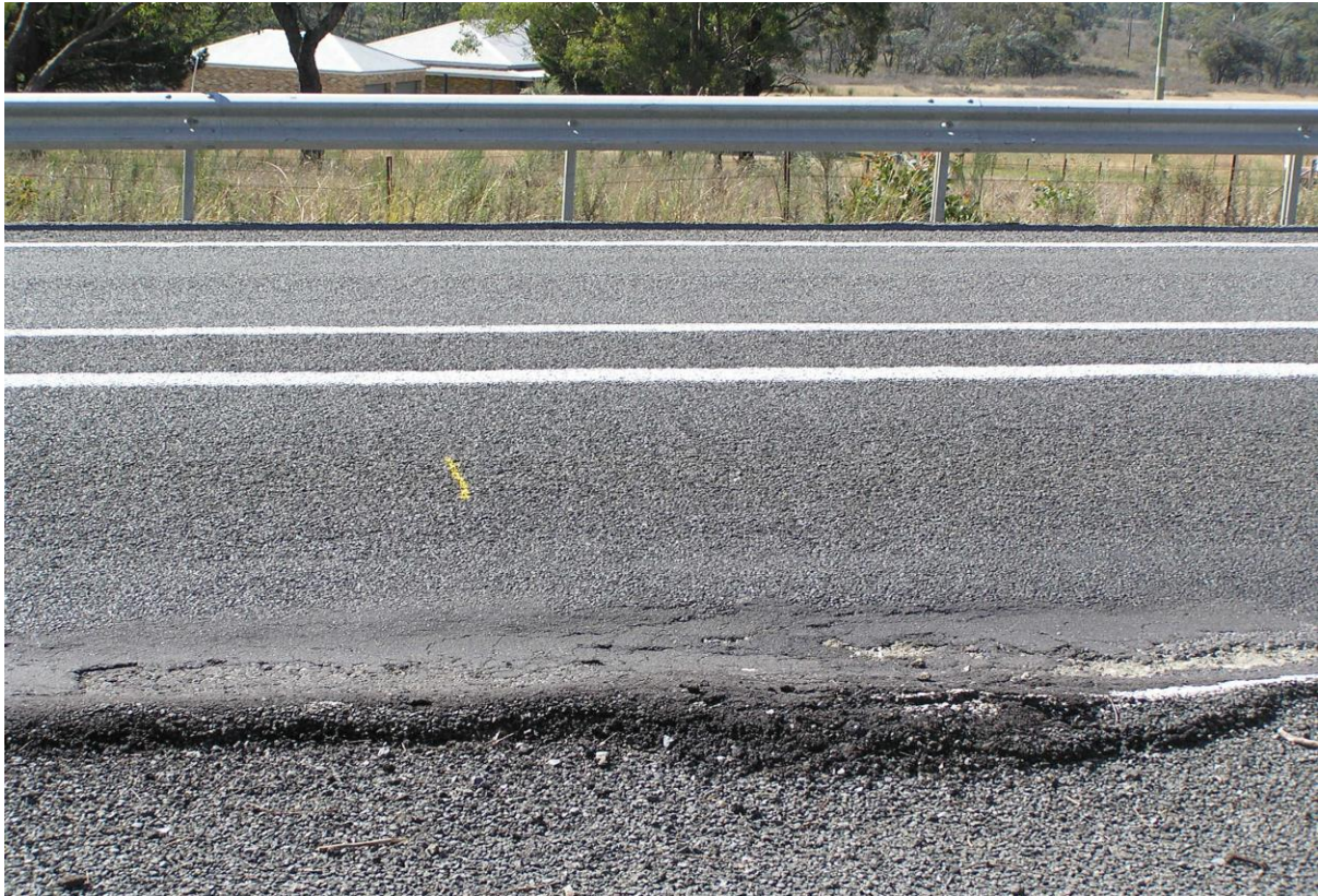
Photo #18_Example of damage close to residence_18Apr21
