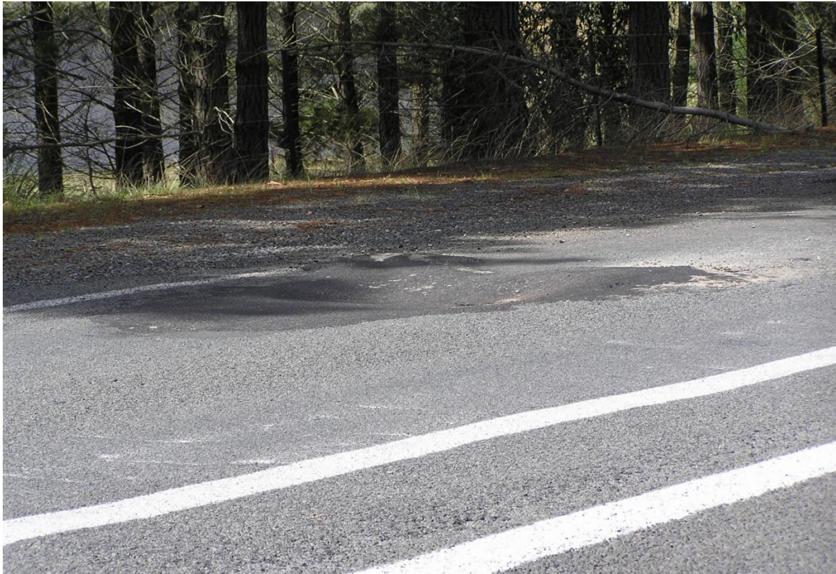
Photo #37 – Large pothole – Ambrose Road (Red Hills Road) approach to Hume Highway_Oct 2021
