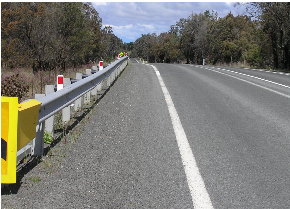
Photo #33 – Corrugation (evident in fog line) along length of Brayton Road producing rolling ‘thunder-like’ noise_Oct 2021
