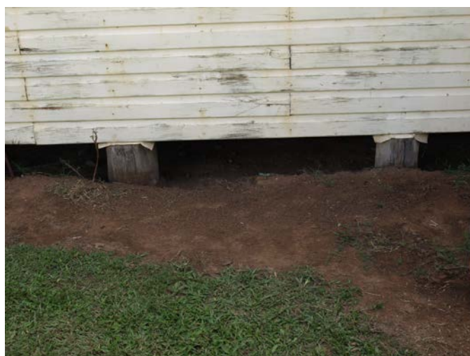
Figure 5. Timber stumps are still serviceable. Ant caps are in place. Soil levels have been built up in order to divert water from beneath the building.
