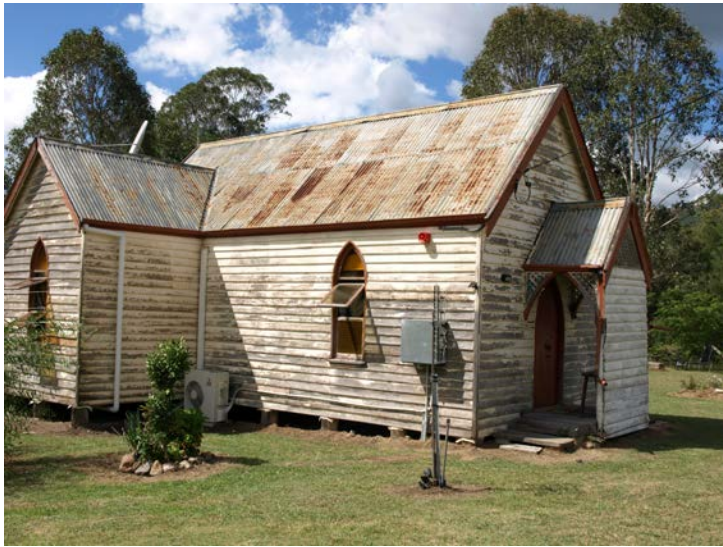
Figure 6. Roofing is in short sheet lengths, some corrosion but in serviceable condition. Cleaning down and anti corrosion treatment would be necessary. Walls require some repairs and cleaning down of old lead paint and sanding prior to priming and recoating
