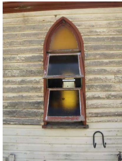
Figure 7. Windows are serviceable, but in need of some glazing repairs and replacement as well as reputtying using traditional linseed putty
