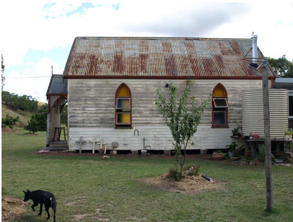
Figure 8. East Elevation showing the general condition of the exterior. Water tanks are new and plumbed into the guttering.
