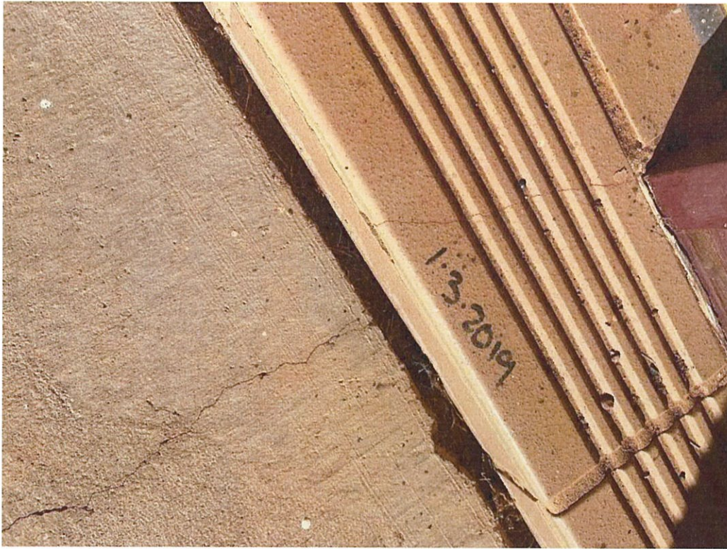
Figure 27: Front Verandah/tiles at front door, cracking in concrete/tiles
