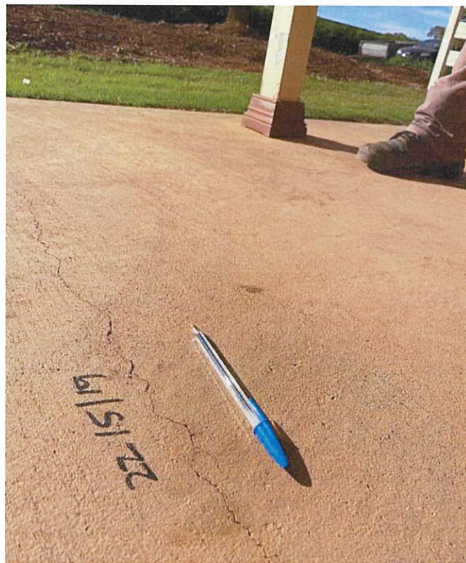
Figure 26: Front Verandah, cracking in concrete
