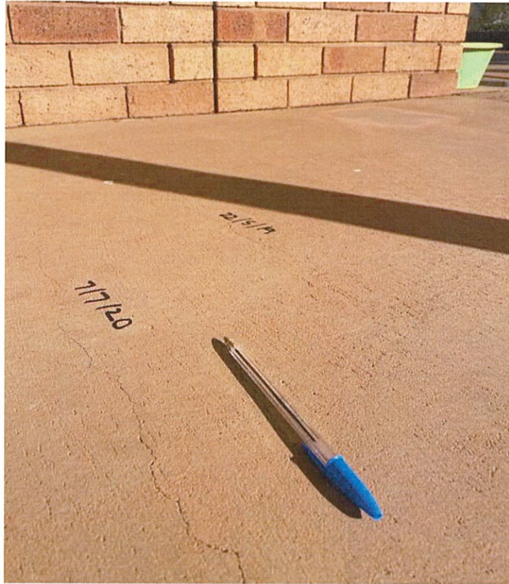
Figure 25: Front Verandah, cracking in concrete
