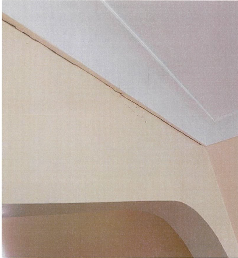
Figure 13: Front door foyer, crack above archway
