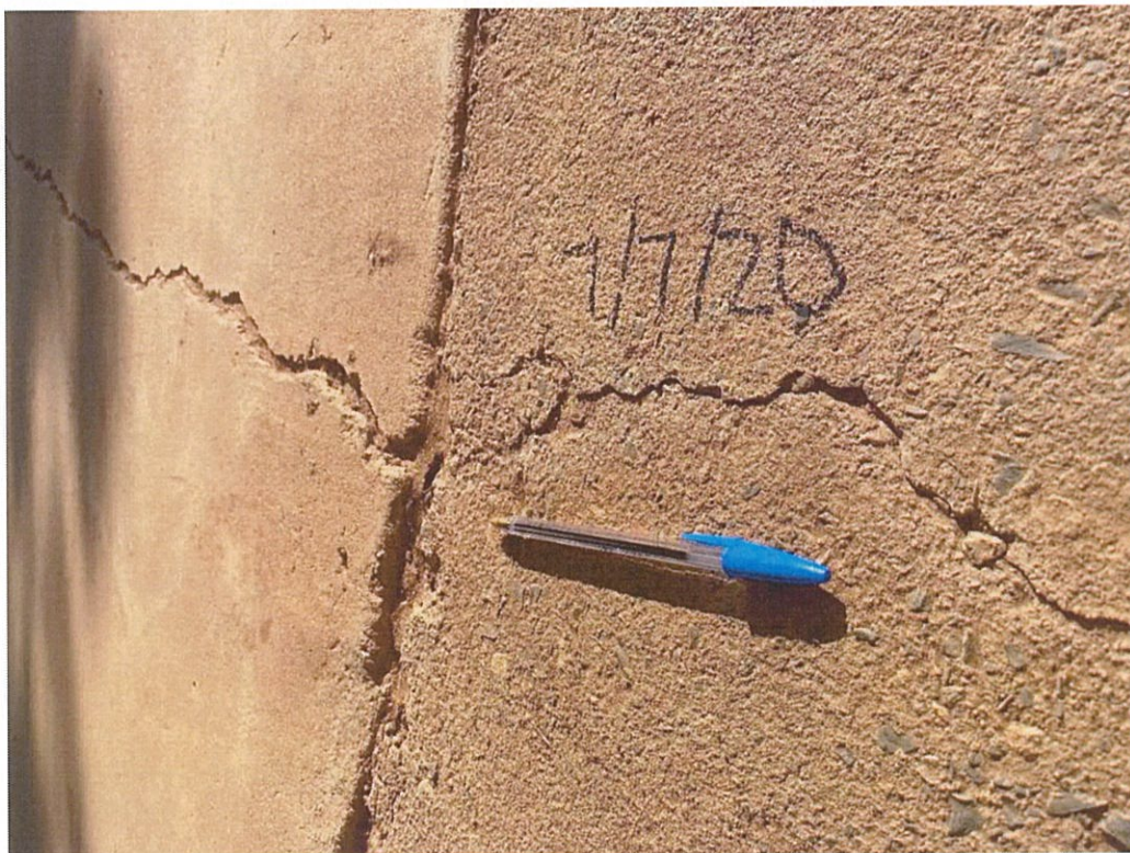
Figure 24: Carport/Verandah, cracking in concrete
