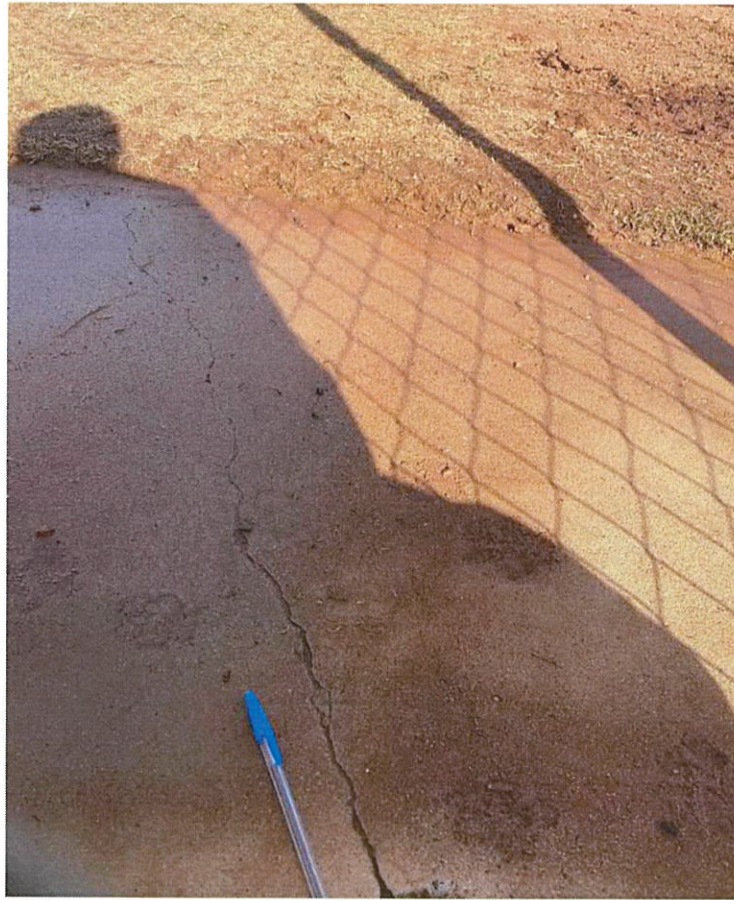
Figure 21: Carport leading to backyard, cracking in concrete
