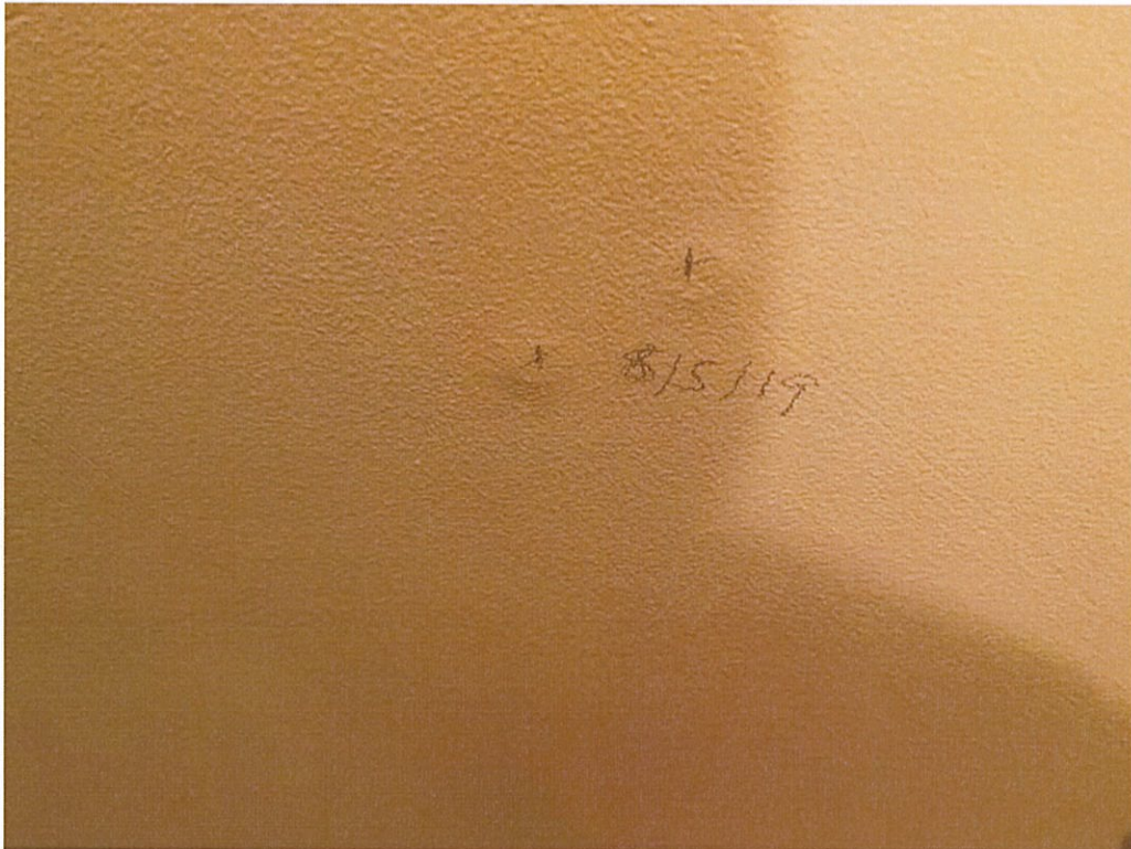
Figure 10: Loungeroom, nails protruding through wall
