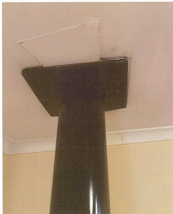
Figure 8: Loungeroom, plate around chimney flue
