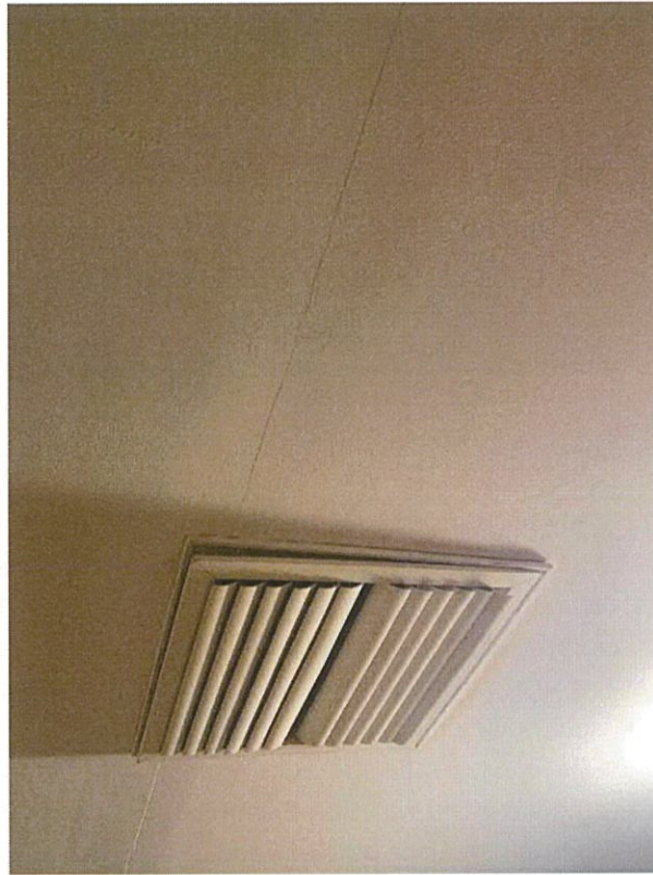
Figure 1: Bedroom 2, air conditioner vent loosened and crack present
