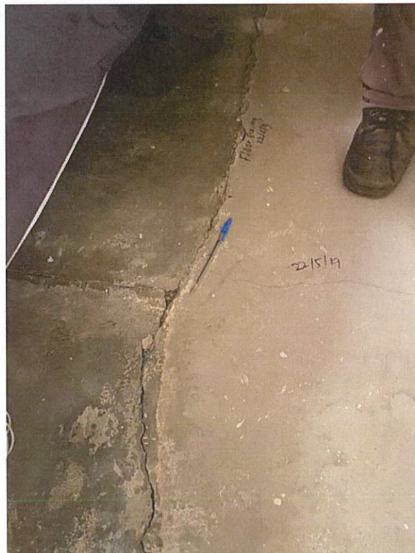
Figure 2: Bedroom 3, Floor Cracking
