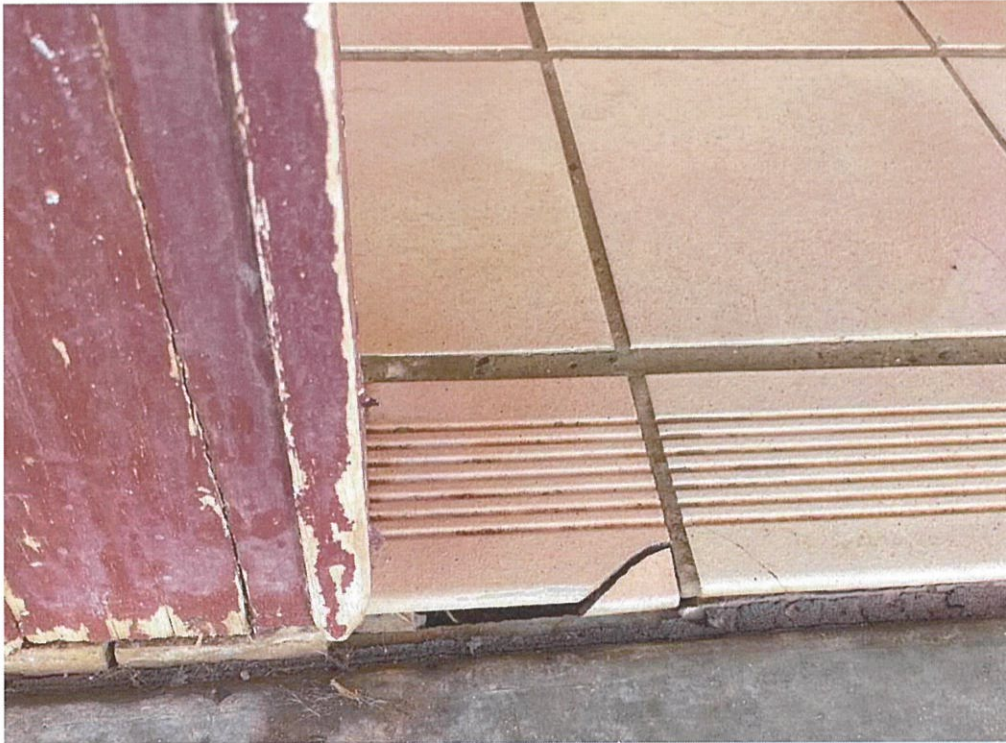
Figure 19: Outside area, broken tile
