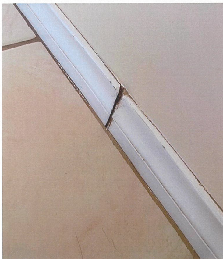
Figure 12: Front door foyer, gap in skirting board
