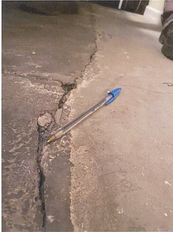
Figure 3: Bedroom 2, Concerns of floor lifting
