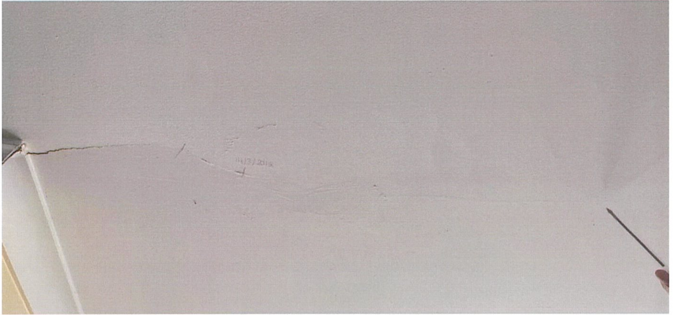
Figure 15: Kitchen, crack in roof
