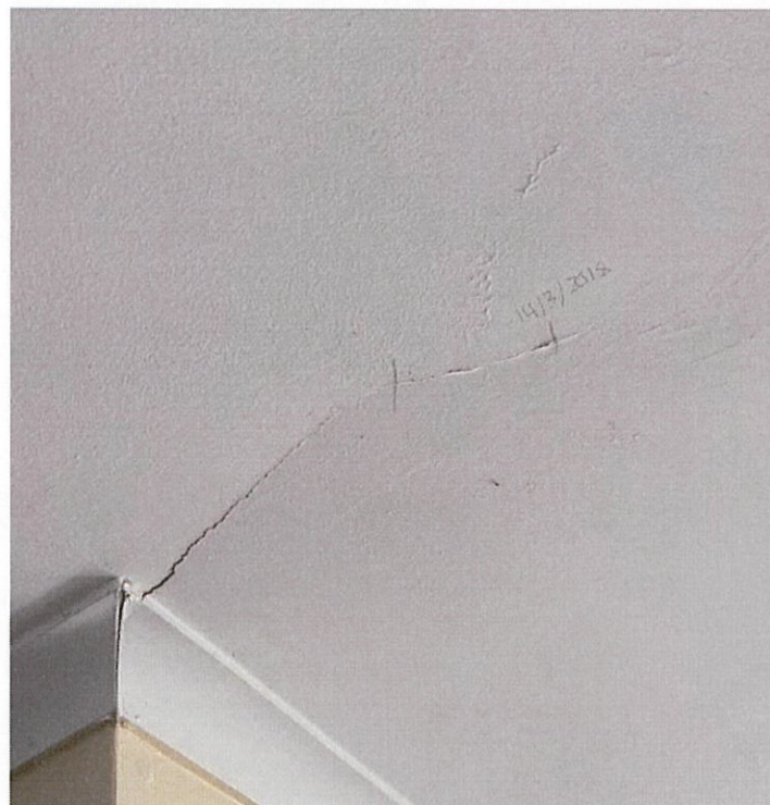
Figure 14: Kitchen, crack in roof
