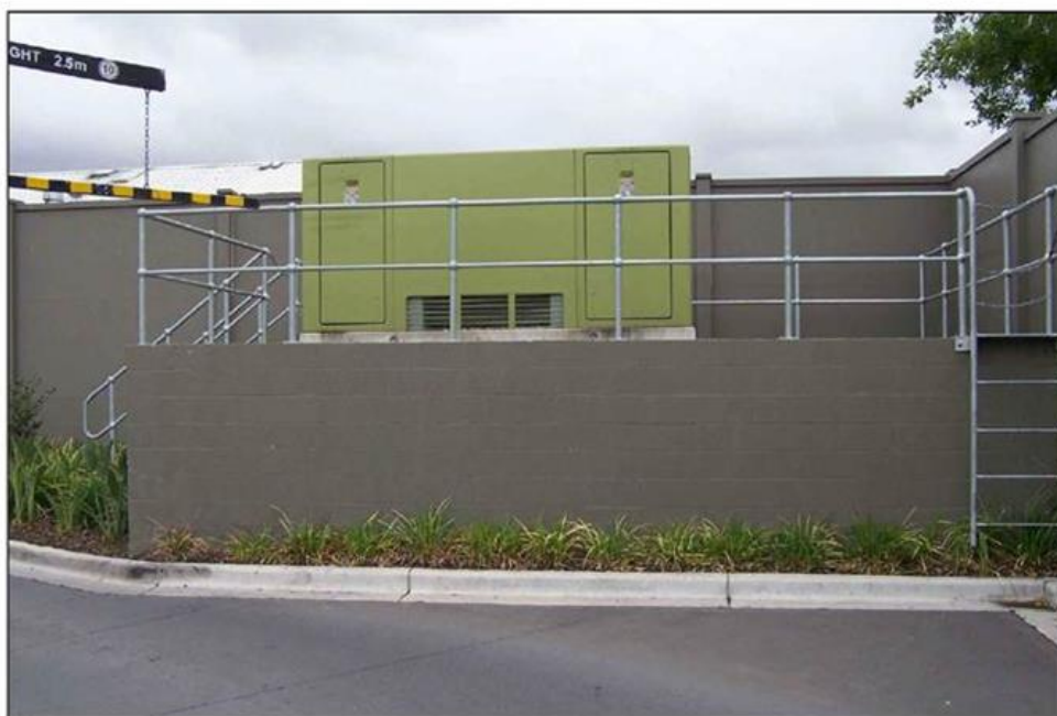
Figure 51 - Example substation raised above 1:100 flood level
