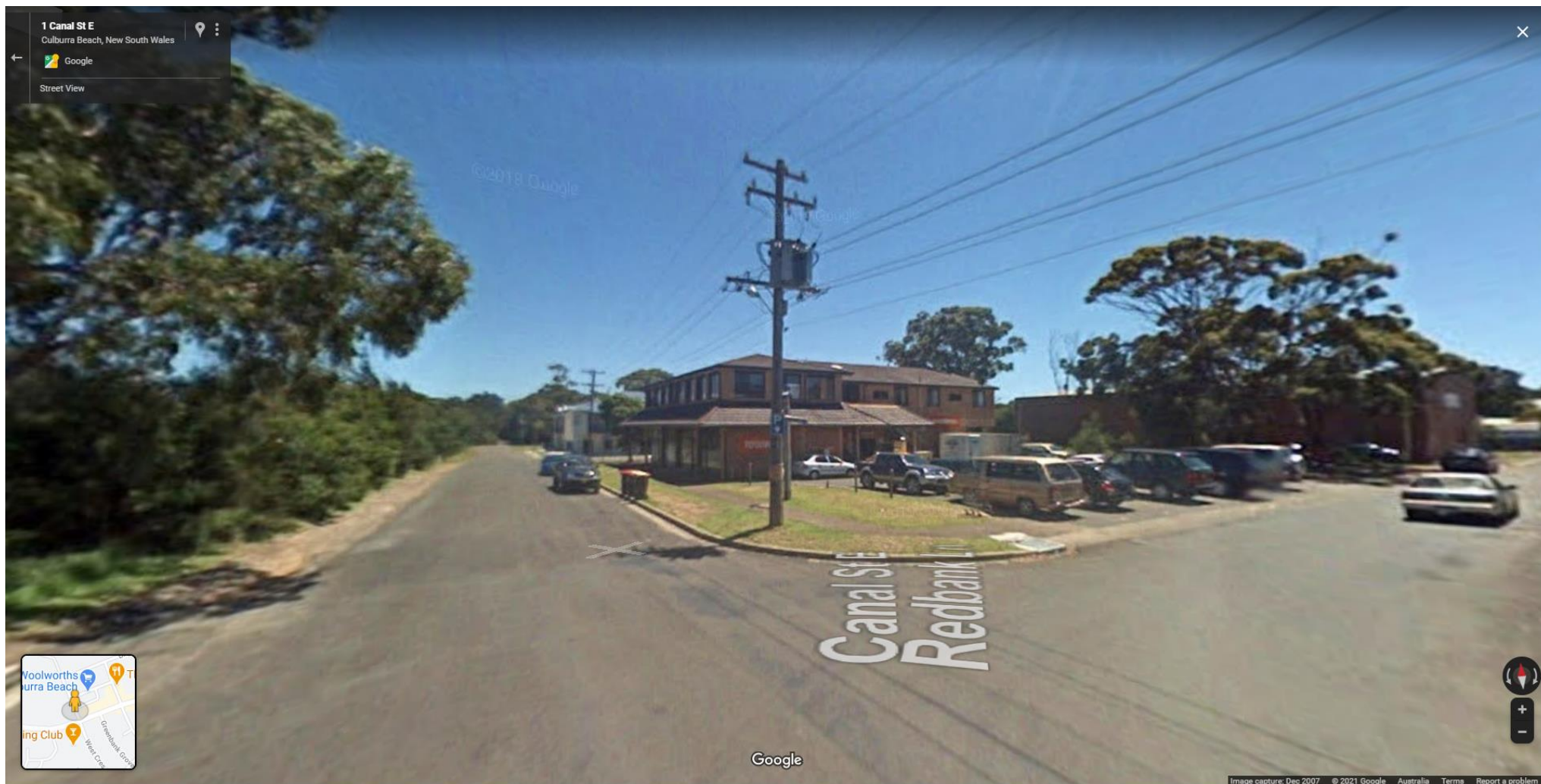
Low voltage and 11 kV high voltage overhead power in Canal Street East showing pole mounted substation no. 51602.
