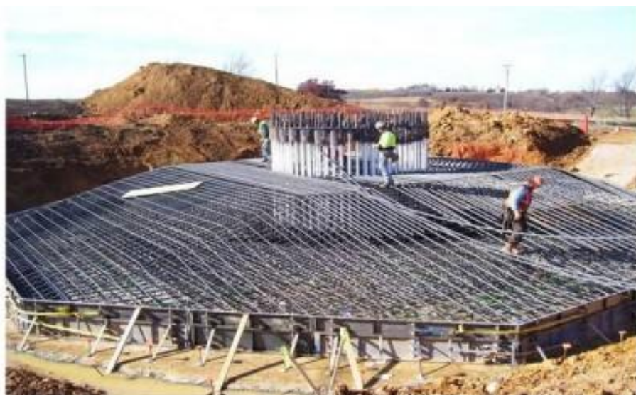
A single wind turbine concrete base under construction
