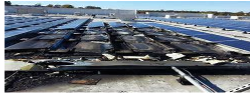
Fire damage to a PV solar IEGW
