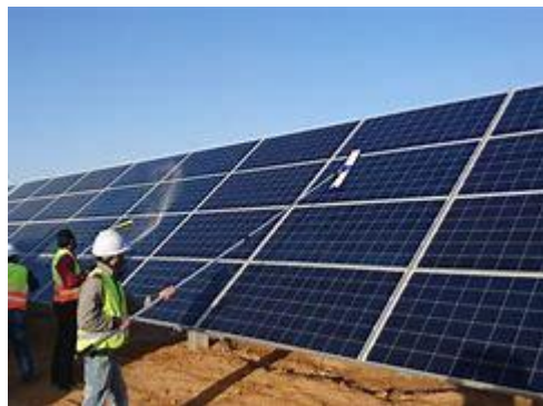
Cleaning PV solar panels
