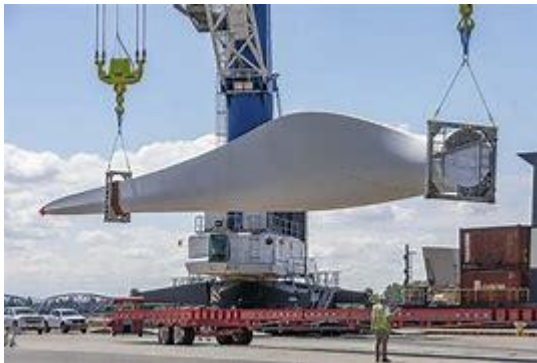
Unloading a wind turbine blade from a ship
