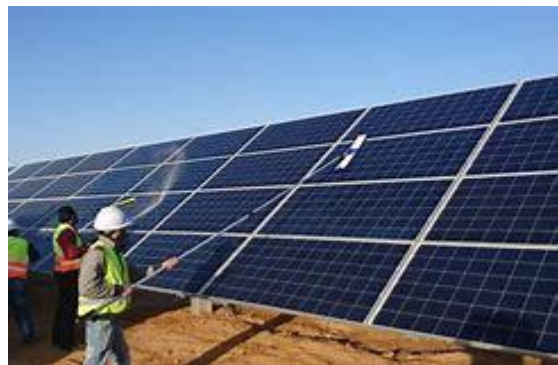
Cleaning PV solar panels
