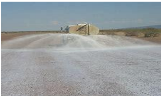
Construction site dust control
