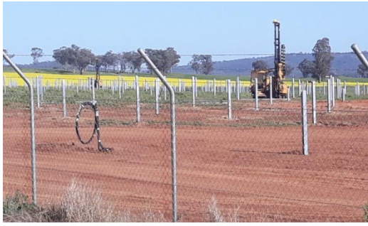
Land cleared. cables laid. pile-driven uprights in place
