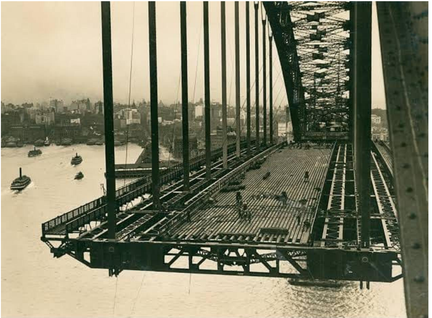
Figure 3.3.5.6 – Harbour bridge heavy trusses to support trains both sides
