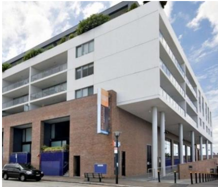
Photos showing structural columns supporting overhanging upper levels
