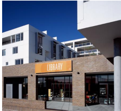
Photos showing structural columns supporting overhanging upper levels
