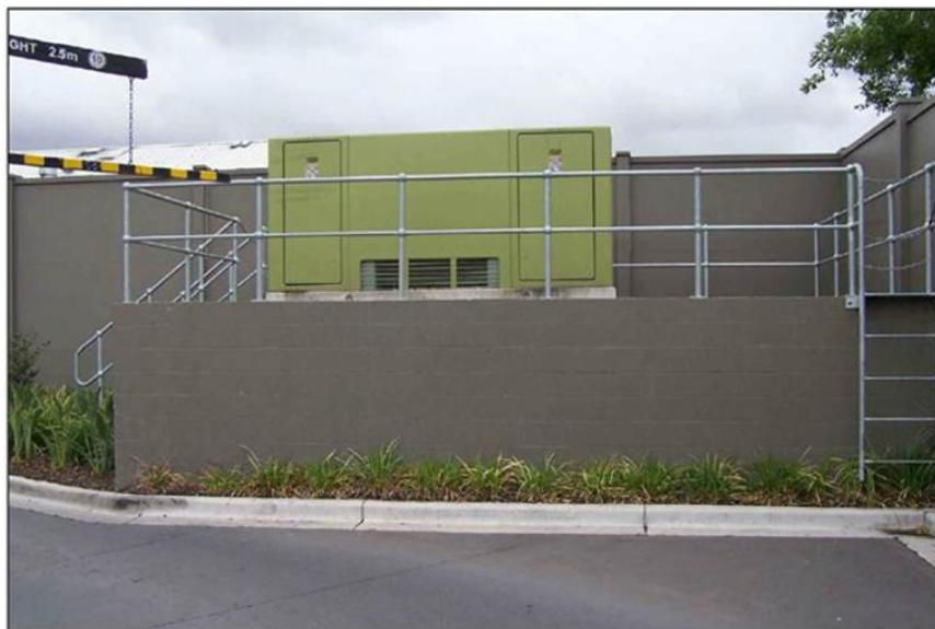
Figure 51 - Example substation raised above 1:100 flood level
