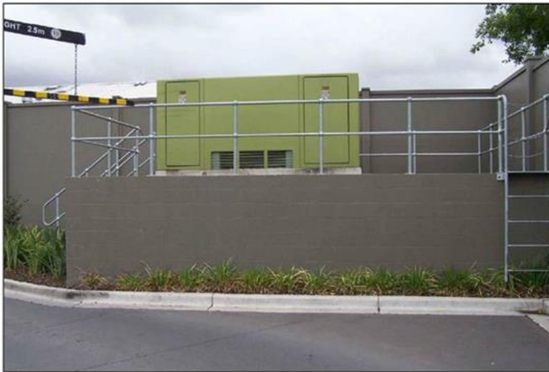
Figure 51 - Example substation raised above 1:100 flood level
