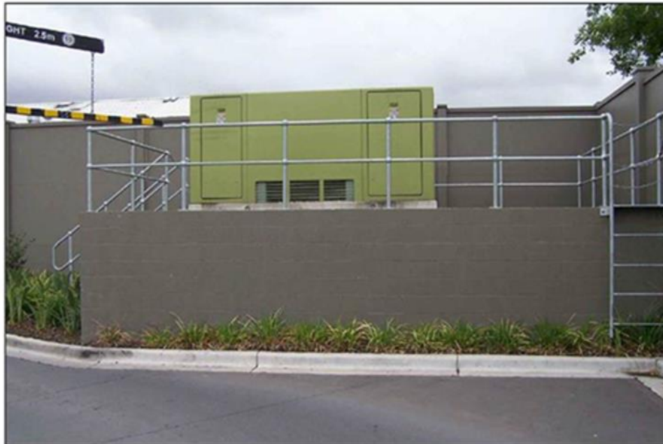
Figure 51 - Example substation raised above 1:100 flood level
