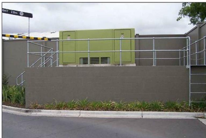
Figure 51 - Example substation raised above 1:100 flood level
