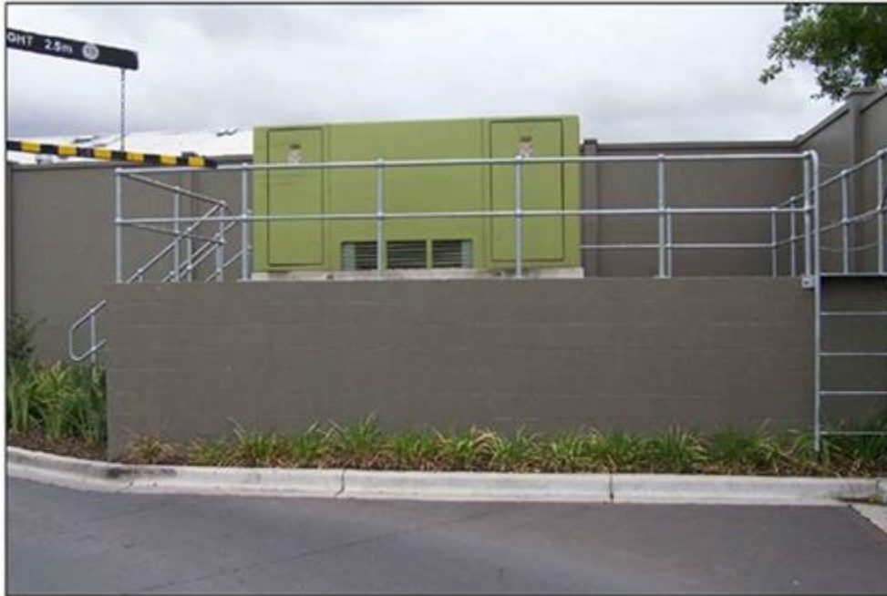
Figure 51 - Example substation raised above 1:100 flood level
