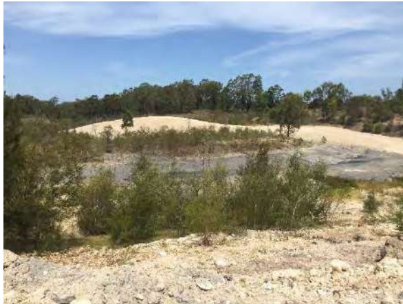
Photograph 43. Former water body in centre of Lot 7314 (noted in previous inspection as having been drained) – channel cut to prevent future ponding. The large carbonaceous material stockpile and outcrop (in background) covered with sandstone fill (presumably sourced from the site, but not confirmed). View southeast.
