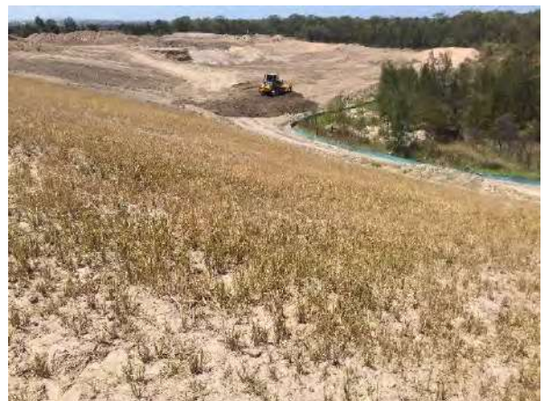
Photograph 20. Embankment in eastern portion of Part Lot 401, recently excavated to rock, top-soiled and seeded (as noted in Section 0). View northeast.
