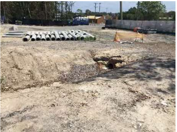
Photograph 4. Unlined channel and concrete pipe culvert under access track. Metford Road gate in background. View southwest.
