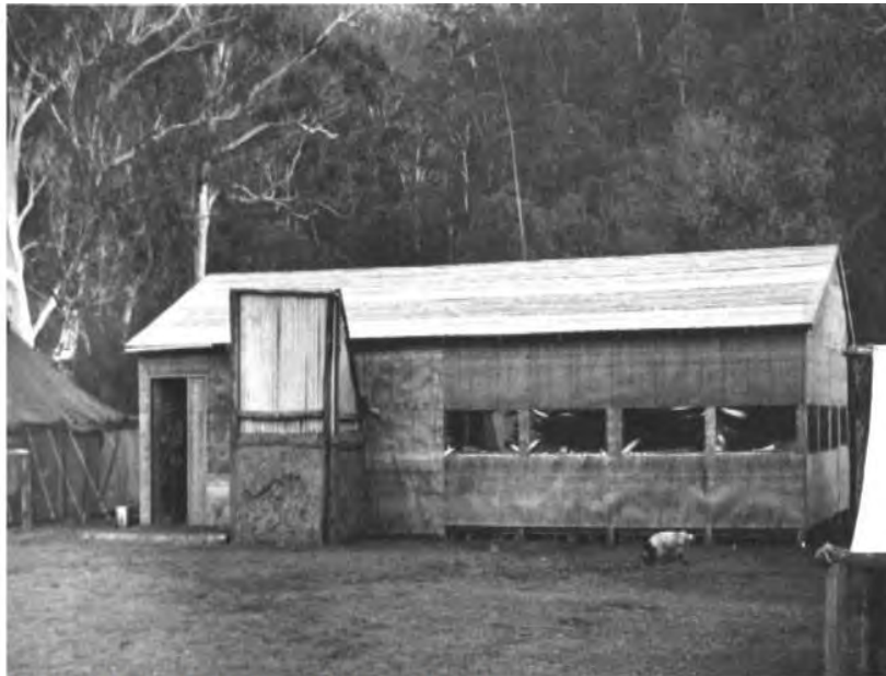
Lobs Hole drawing Office, 1951. Building clad with “Malthoid” paper, using transparent drawing paper as glass windows. SMA Photo
