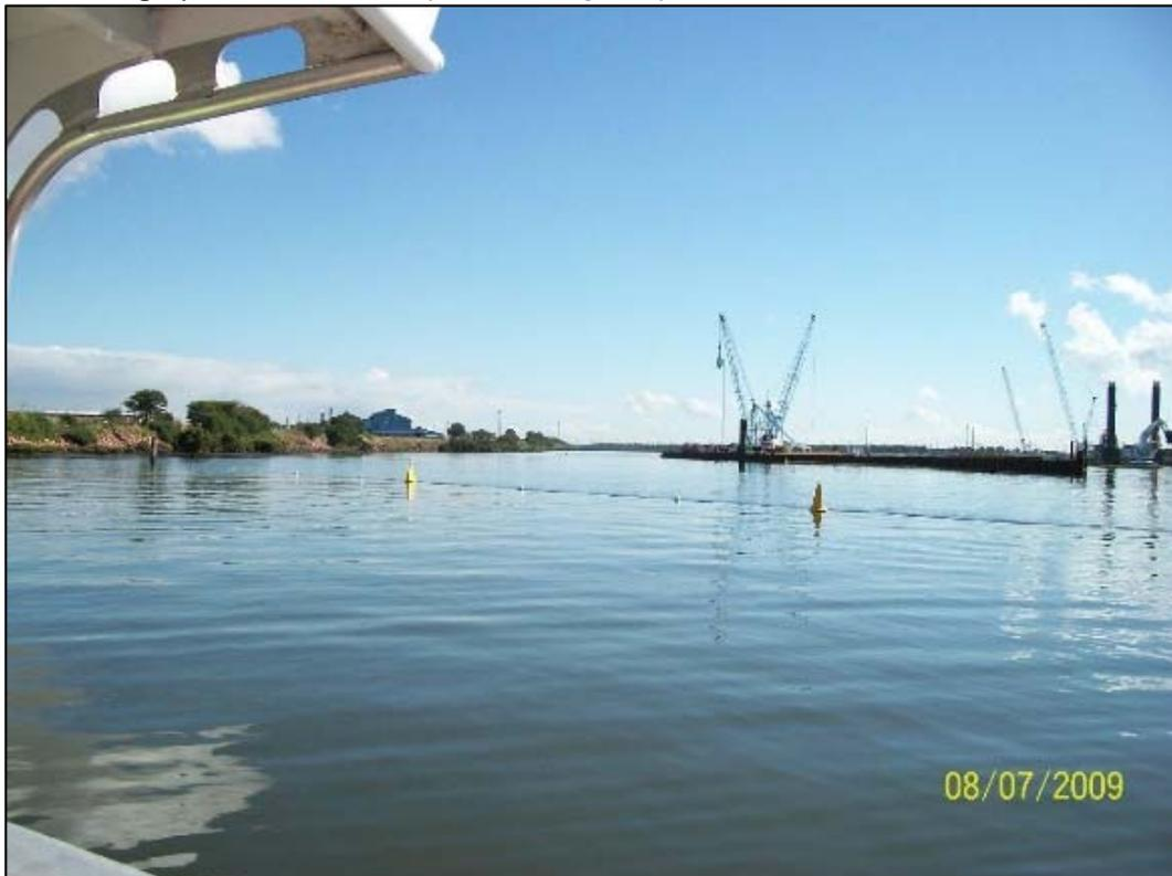
*Photograph 3. Silt Curtain in place*
