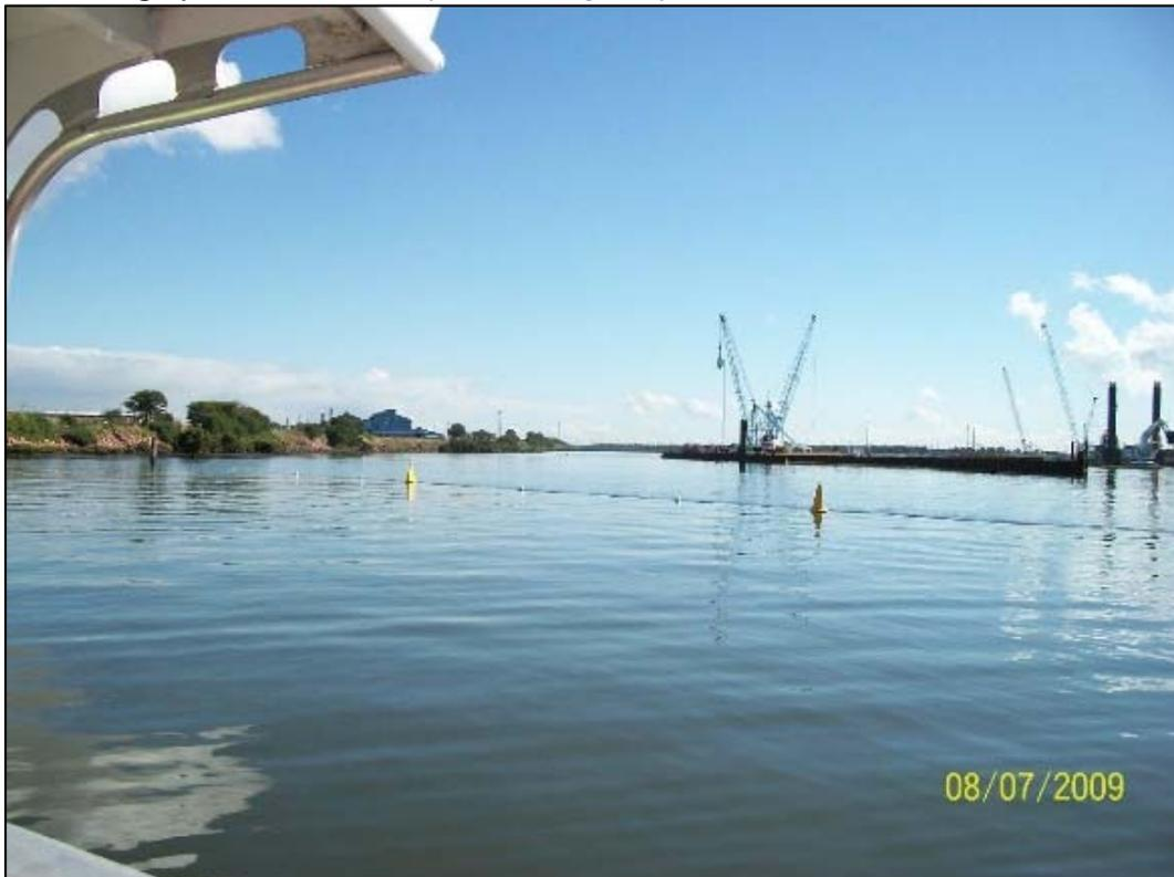
*Photograph 3. Silt Curtain in place*
