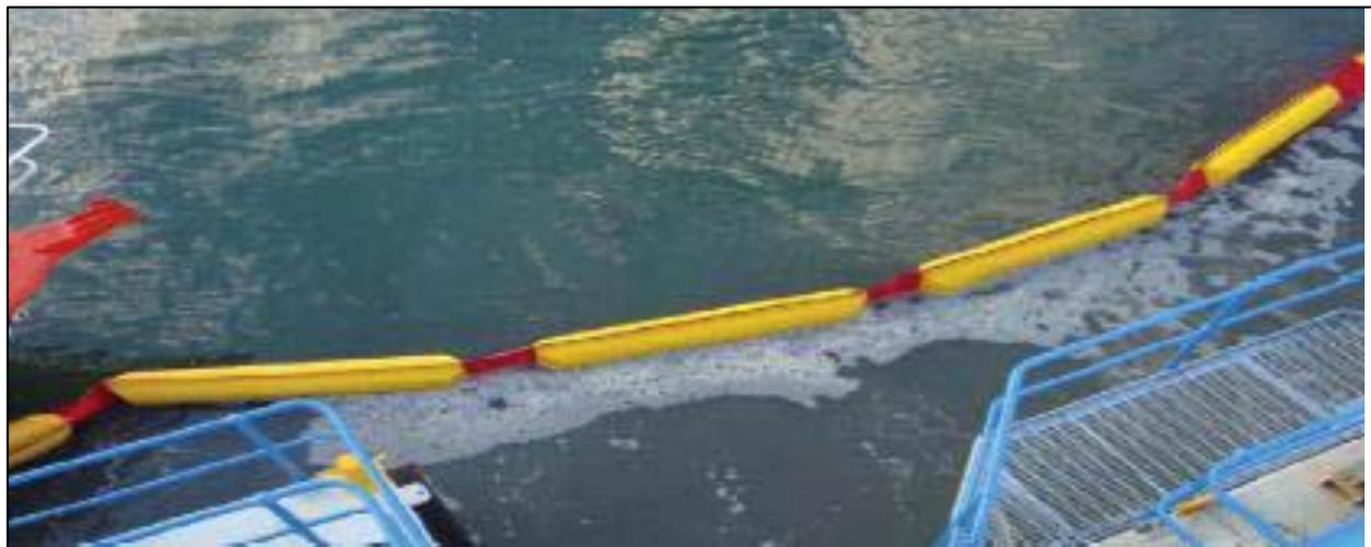
**Figure 5 Silt Curtain to deployed around dredging and disposal works areas**
