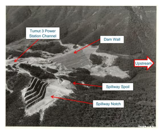
Figure 16: Historic photograph from construction of Talbingo Reservoir (3 September 1970).
