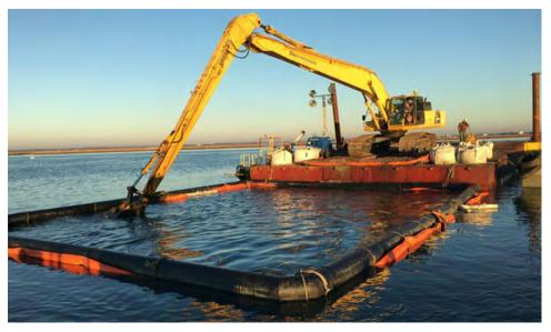
Figure 24: Example construction barge and excavator operating within a 'moon pool' (floating silt curtain).
