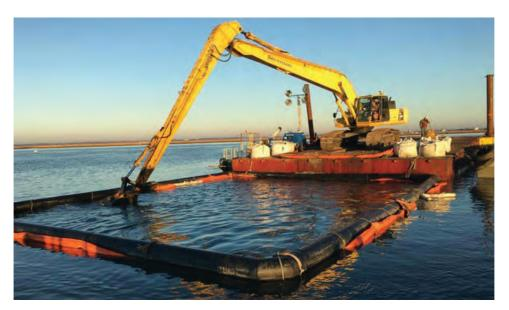
A combination of on-land placement and subaqueous placement of the dredge material is proposed.
