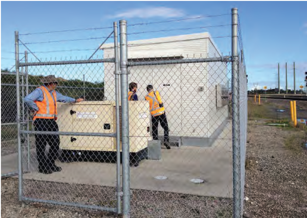
Plate 10 Indicative design of signalling location hut to be installed within the study area (note the signalling hut will not be fenced as it will be located within the fenced rail corridor)
