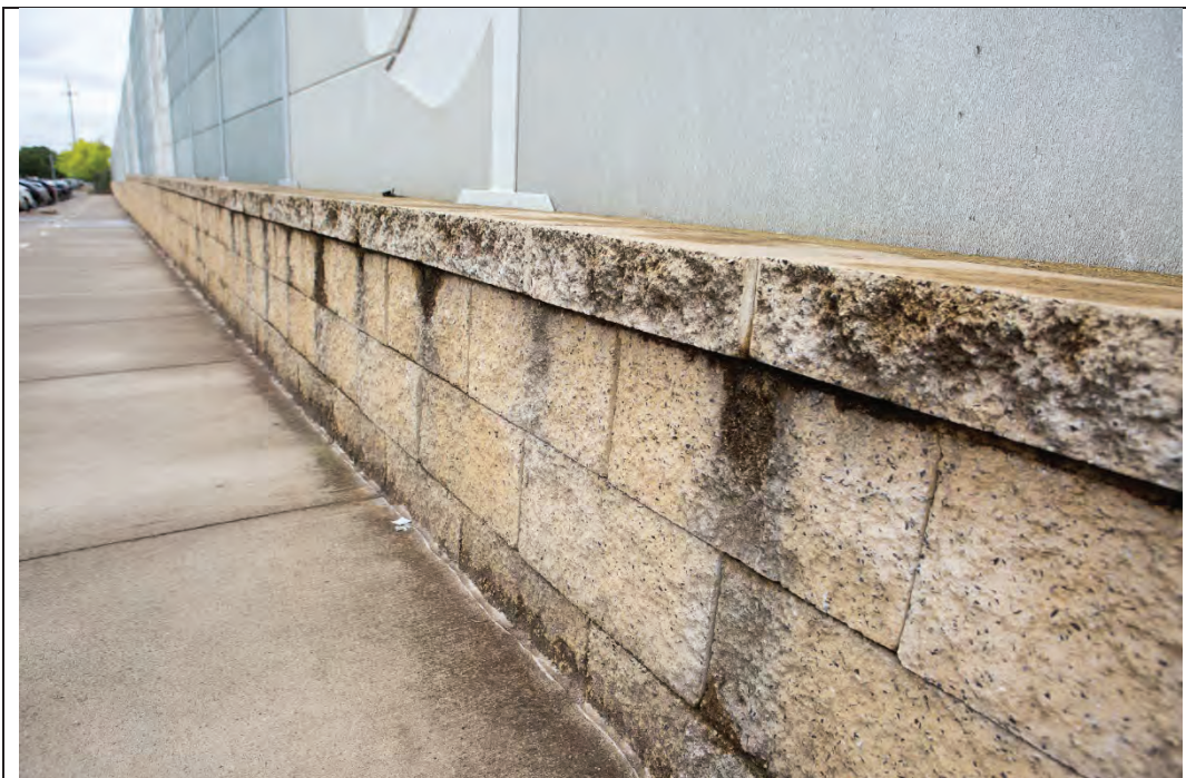
Photo 3: Concrete buffer wall, with concrete aggregate brick retaining wall
