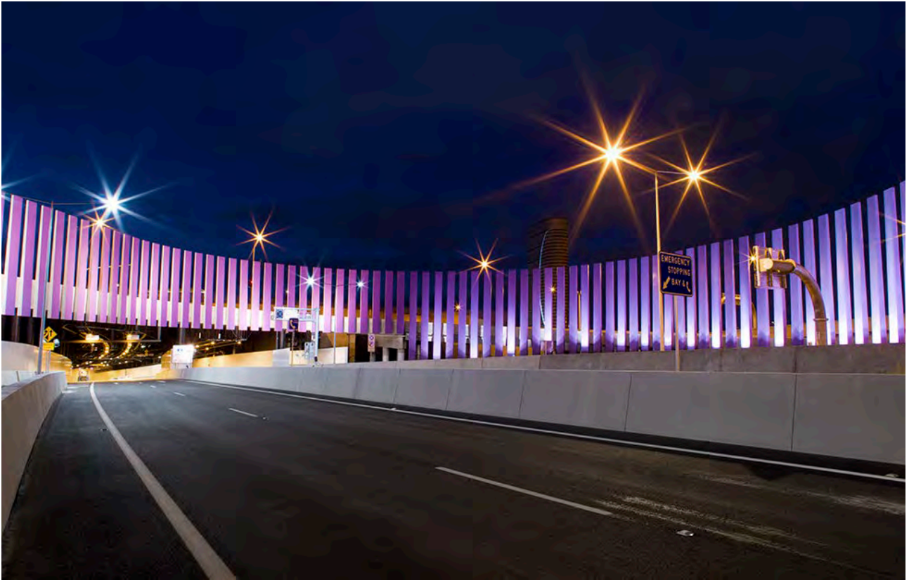
Figure 5-12: Tunnel portal design example - Airport Link M7 tunnel portal entry in Brisbane provides a distinctive tunnel entry experience with minimal road furniture and clutter to distract the driver experience
