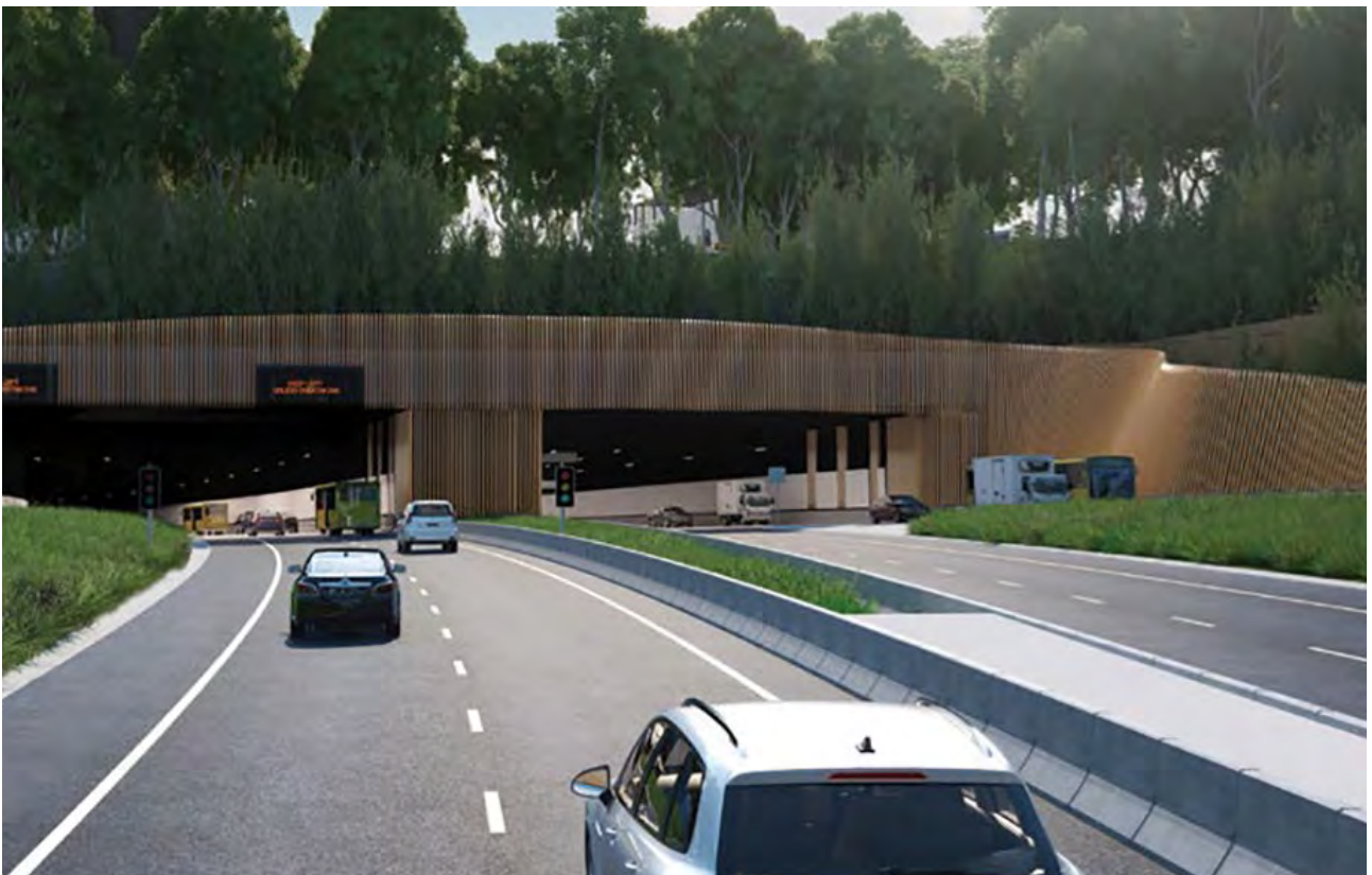
Figure 5-13: Tunnel portal design example - the tunnel portal entry experience should include organic forms to integrate with the surrounding landscape setting of the Rockdale Wetlands
