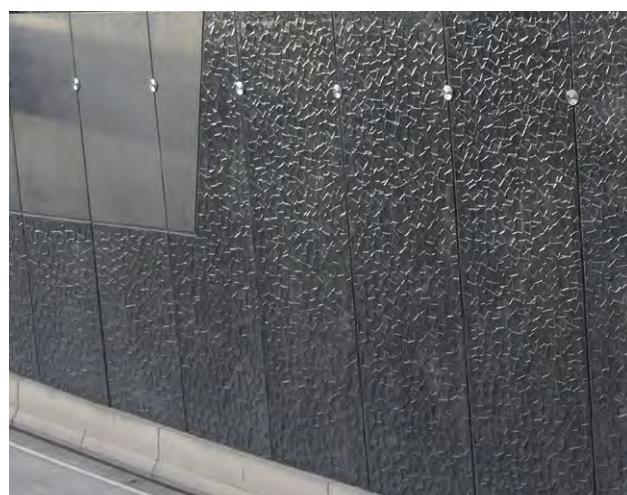
Figure 5-9: Colour treatment examples - colours complementary to natural concrete and integrated with other structural elements.
