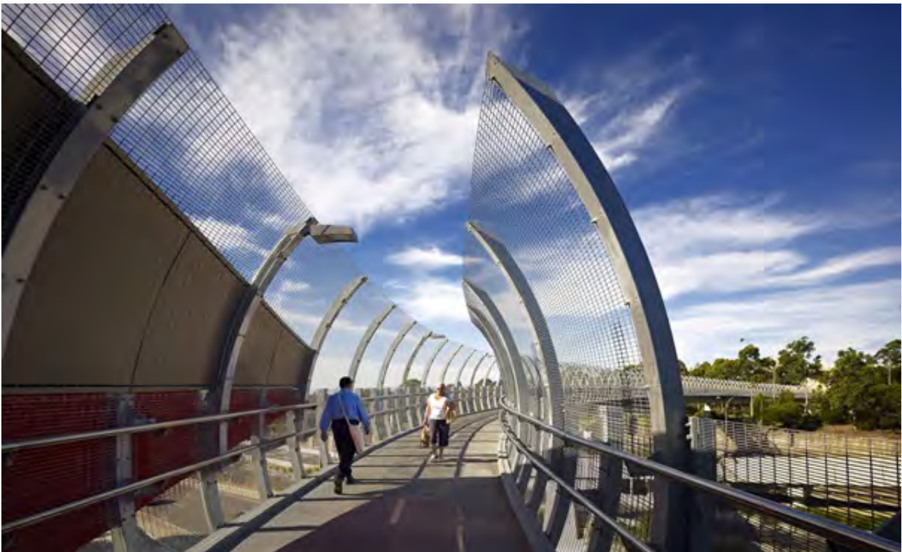
Figure 5-32: President Avenue shared cycle and pedestrian bridge design example - All bridge components including throw screens, lighting and fencing need to be considered as part of the overall composition of the bridge
