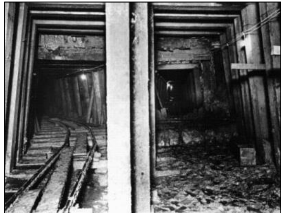
Figure A.13.4: Timbered tunnel 1929 (Source: Sydney Water Corporation)
