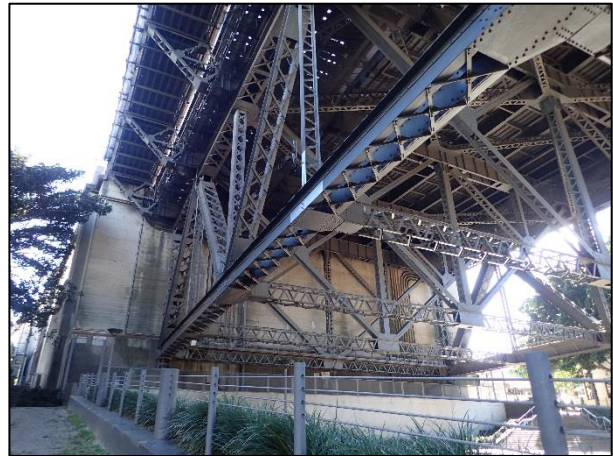
Figure A.8.7 : Steel trusses of the Sydney Harbour Bridge approach span adjoining the concrete arch of the Milsons Point (Fitzroy Street) Underbridge, facing north
