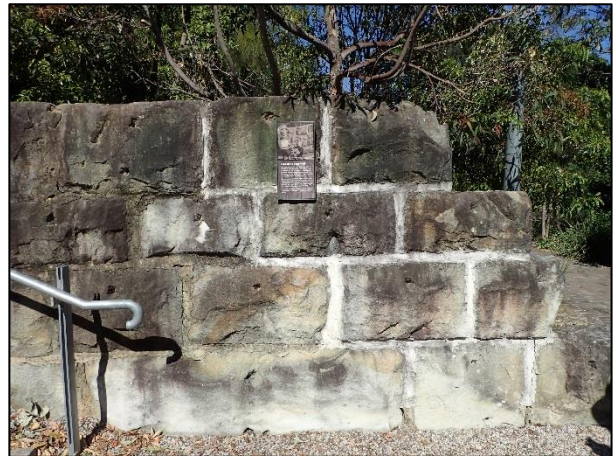
Figure A.5.4 : Part of the sandstone bund wall
