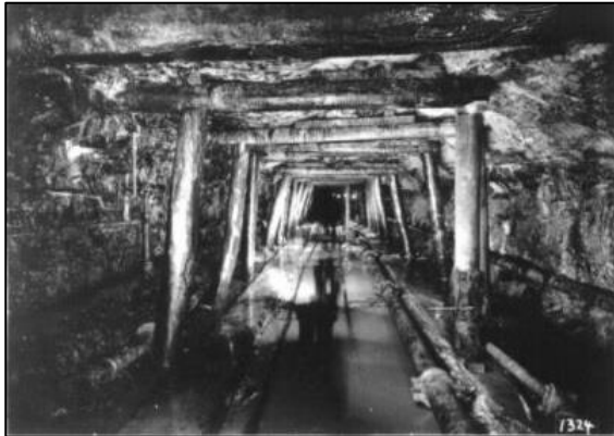
Figure A.13.1 : Tunnelling showing timbered supports of roof 1929 (Source: Sydney Water Corporation)
