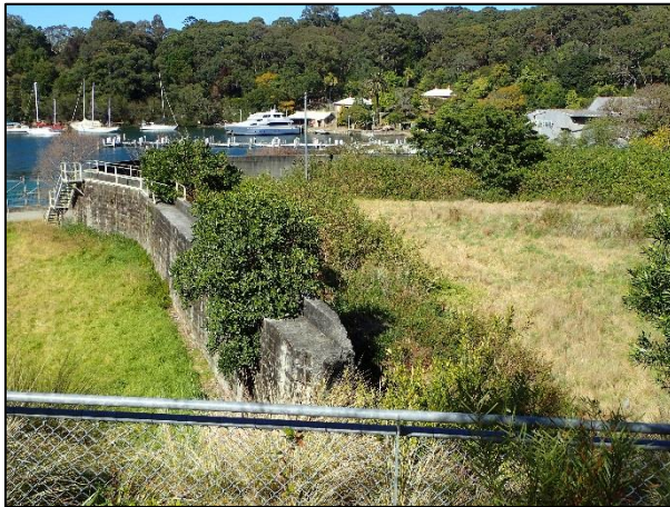
Figure A.7.9 : Bund wall (12) using convict hewn sandstone; Area of Archaeological Potential A to right of wall
