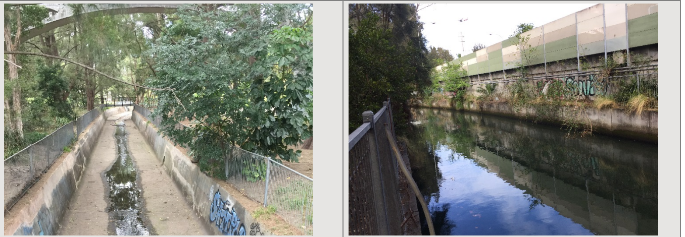
Figure 4-2 Whites Creek concrete-lined stormwater channel. Upstream section (left photo). Downstream section (right photo)
