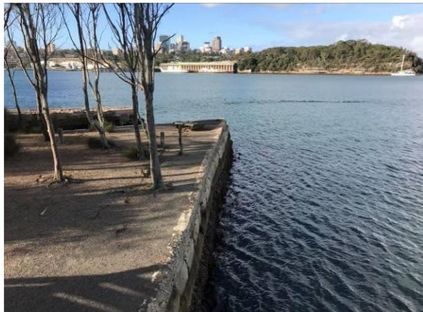
**Plate 8 Sandstone retaining wall at Yurulbin Point construction support site (WHT4)**
