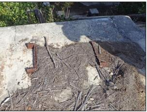
Figure A.12.9 Detail of the rusted metal embedded at the top of the concrete staircase, facing north towards the Bantry Bay Reservoir (WS 0008)
