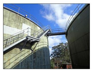
Figure A.12.6 Metal staircase attached to Bantry Bay Reservoir (WS 0008), and catwalk connecting the two Reservoir (WS 0008) with an inspection point in the reservoirs
