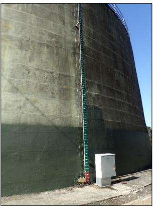
Figure A.12.5 Detail of the water level measure and fuse box attached to the Bantry Bay Reservoir (WS 0008)
