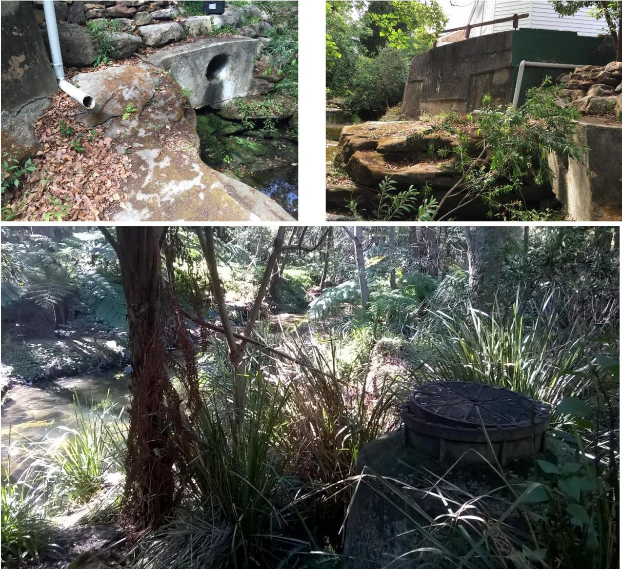
Figure 4-9 Burnt Bridge Creek: concrete stormwater outfalls (top left photo), constructed rock and concrete walls at Kitchener Road crossing (top right photo) and riparian vegetation downstream of proposed culvert showing previous disturbance caused by sewer pipeline and associated pit installation (bottom photo)
