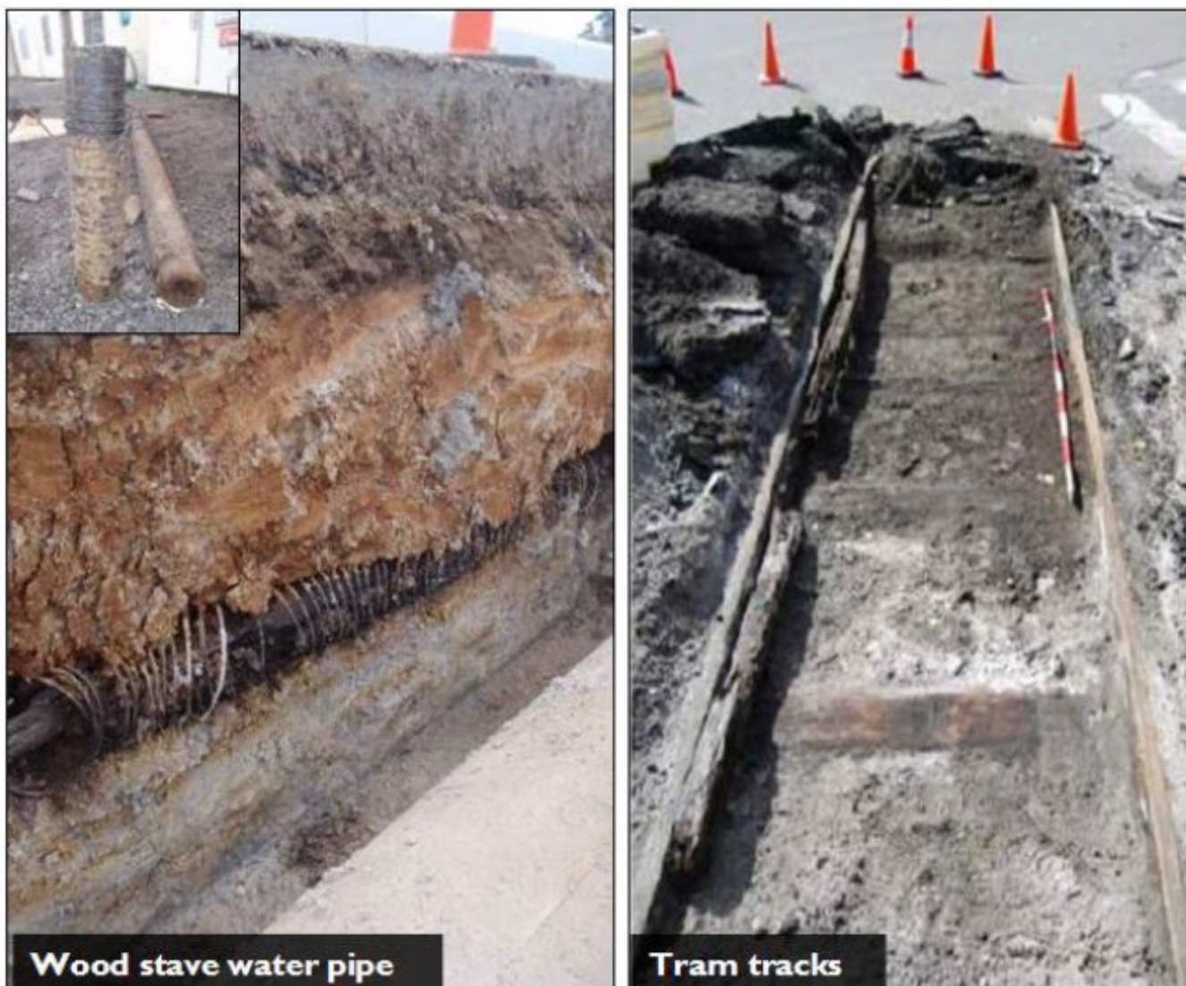
From left to right: Woodstave water pipe with tar and wire sealing (Horsley Drive); Tram tracks (Sydney)
