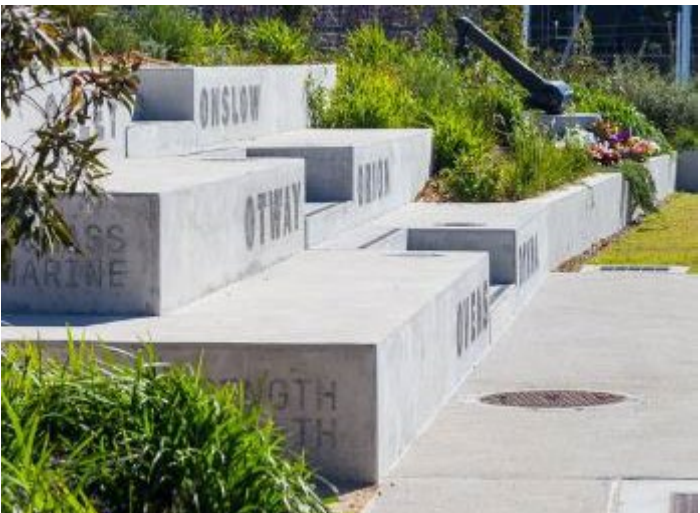
Interpretive text sand-blasted into off-form concrete steps/seats at Sub Base Platypus, Kirribilli. (Source: Urban&Public)
