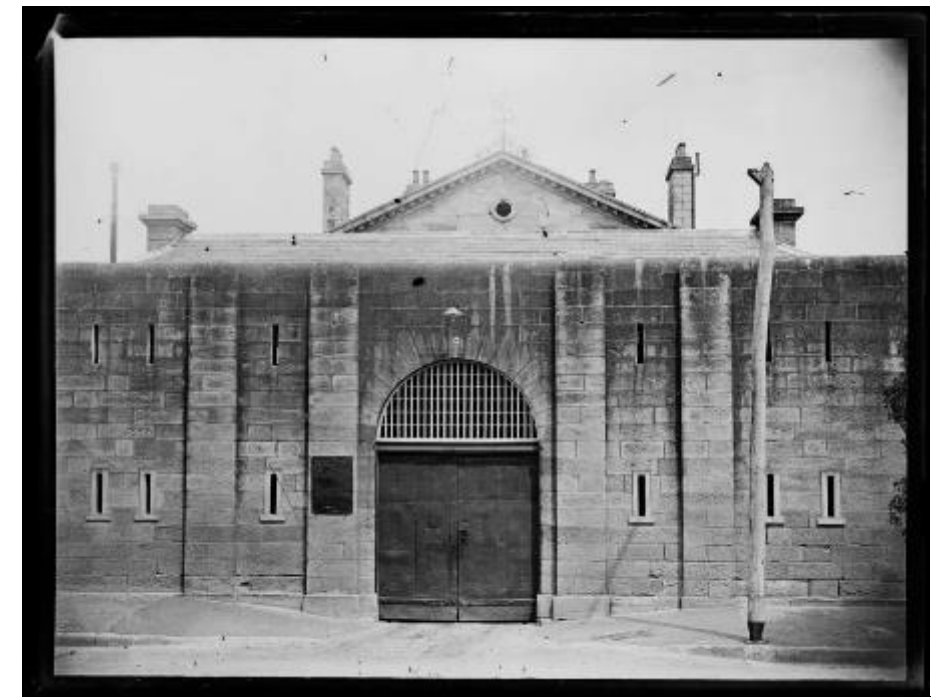
Entrance to Parramatta Gaol, c1930s. (Source: National Library of Australia)
