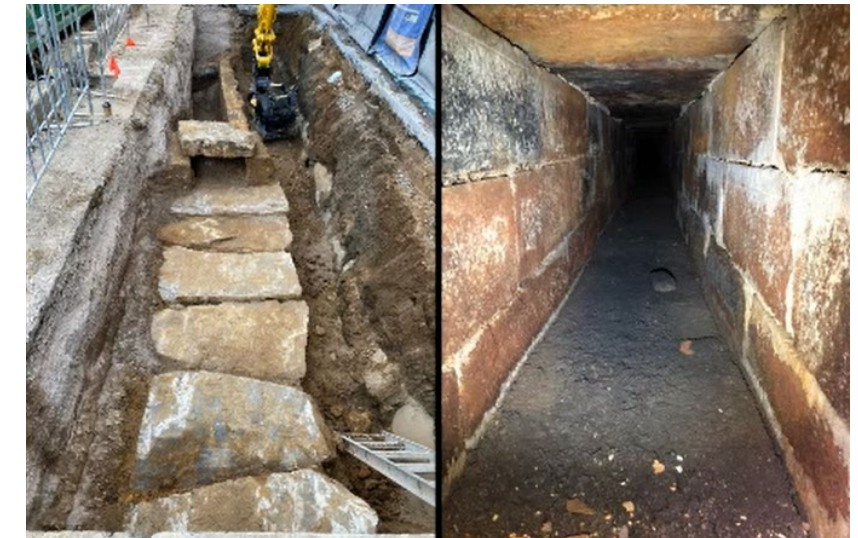
Figure 16 Late 1830s sandstone box drain (Church Street) built at the same time as Lennox Bridge. (Source: GML Heritage)
