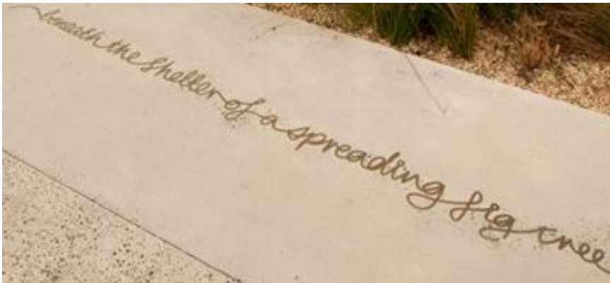
Metallic words inlaid into concrete, Pirrama Park, Ultimo. (Source: Deuce Design)
