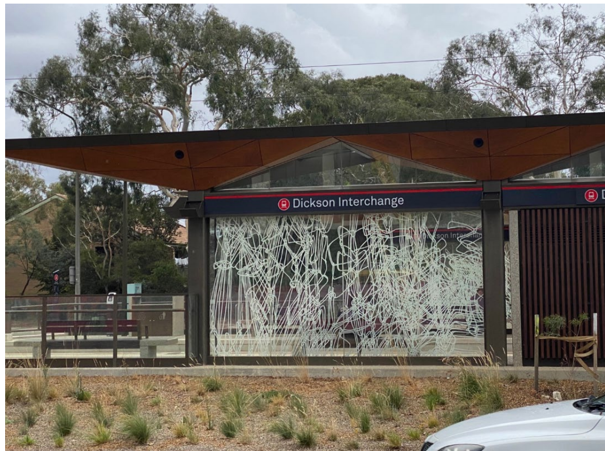
Canberra Metro— stop inlay with heritage design at Dickson Interchange, Canberra (Source: Photo by Gigi Lombardi)
