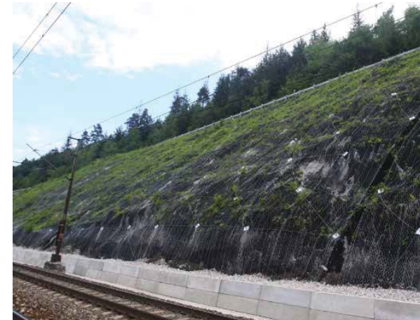
Combination of engineered slopes and low retaining walls to achieve a sculpted land form. Source: COX/HASSELL
