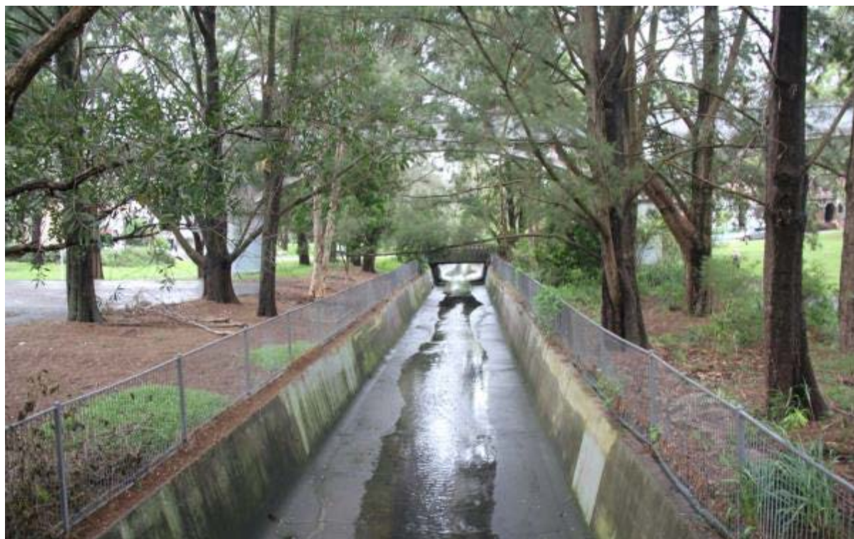
Figure 5-26 The concrete bed of Whites Creek canal looking north from Piper Street bridge
