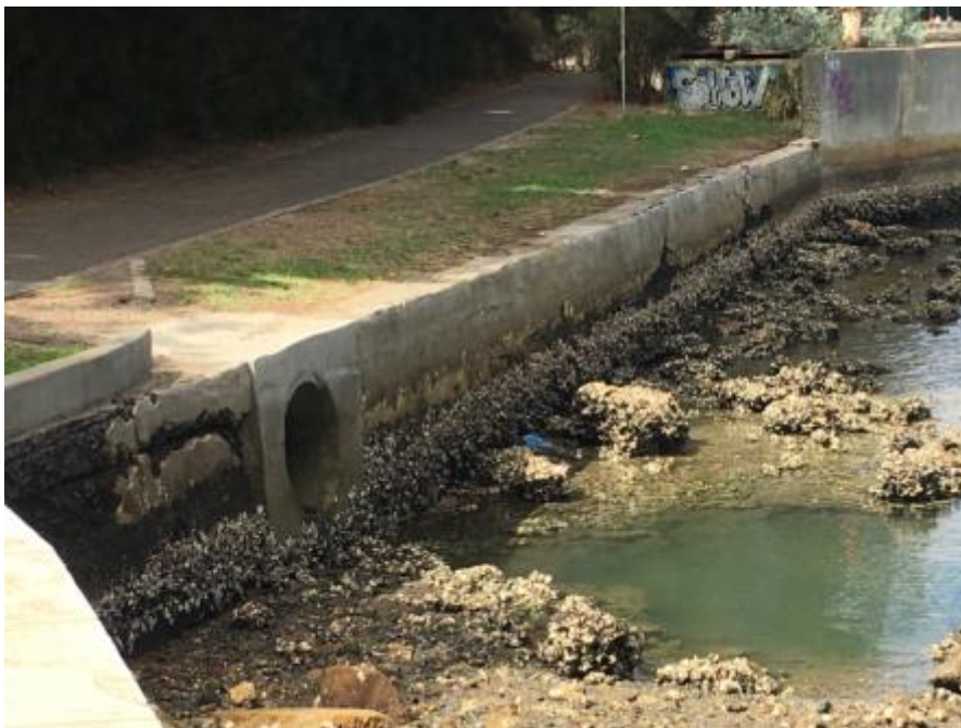
Figure D3-4 Photo of the existing drainage outlet at Iron Cove
