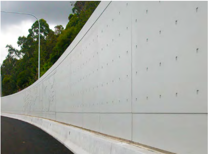
Gore Hill Freeway, Sydney. Provide retaining walls that are topped out by a consistent concrete capping beam. Source: AECOM.
