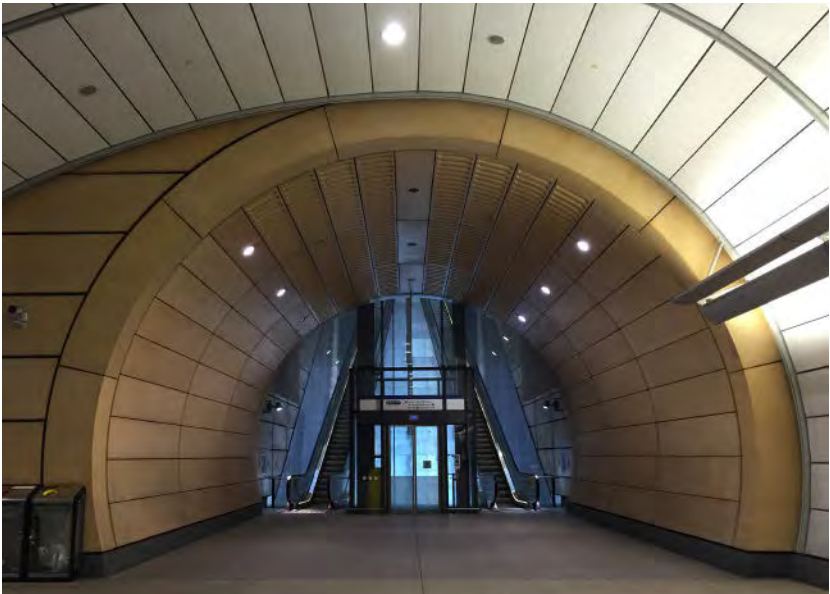
Macquarie Park Station. Services are concealed and integrated within the cavern structure, enabling the clean expression of the cavern form. Architect: Hassell Source: Cox Richardson
