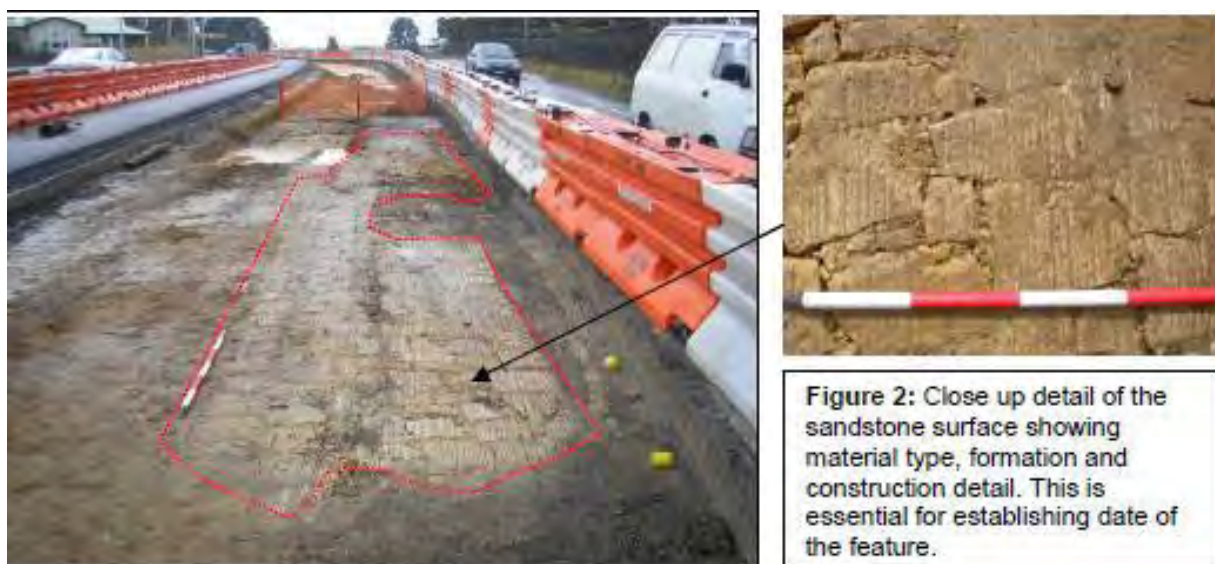
Figure 1: Telford road uncovered on the Great Western Highway (Leura) in 2008 (RMS, 2015).
