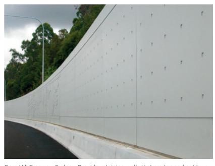
Gore Hill Freeway, Sydney. Provide retaining walls that are topped out by a consistent concrete capping beam.
