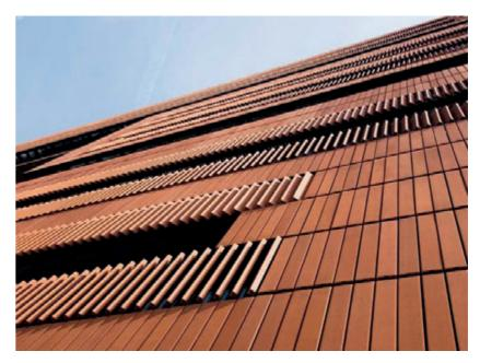
Terracotta louvred facade provides a vibrant wall surface. Source: AECOM.
