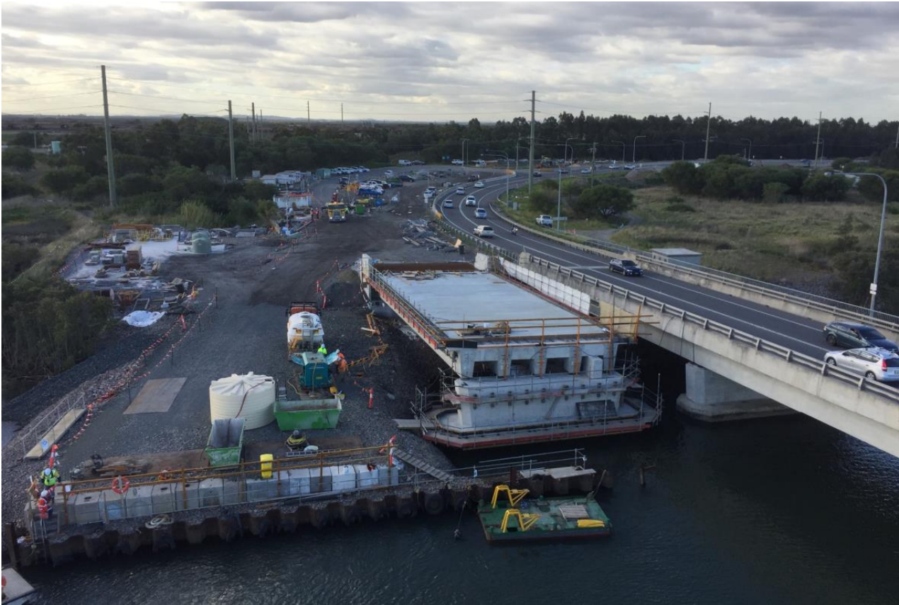
Photo 5-2 Example of a temporary wharf
