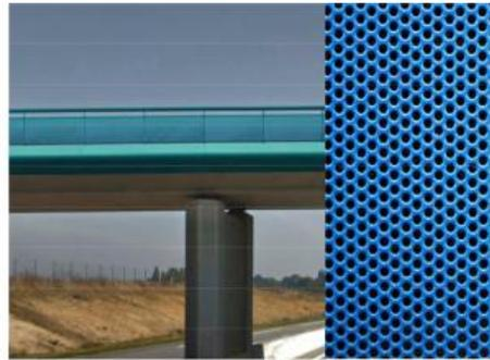
Blue coloured perforated metallic cladding integrated with the safety screen and extending over the bridge parapet of bridges over the M1 Pacific Motorway
