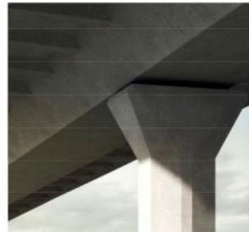
Plain concrete piers with subtle detailing (eg. chamfered or tapered edges)
