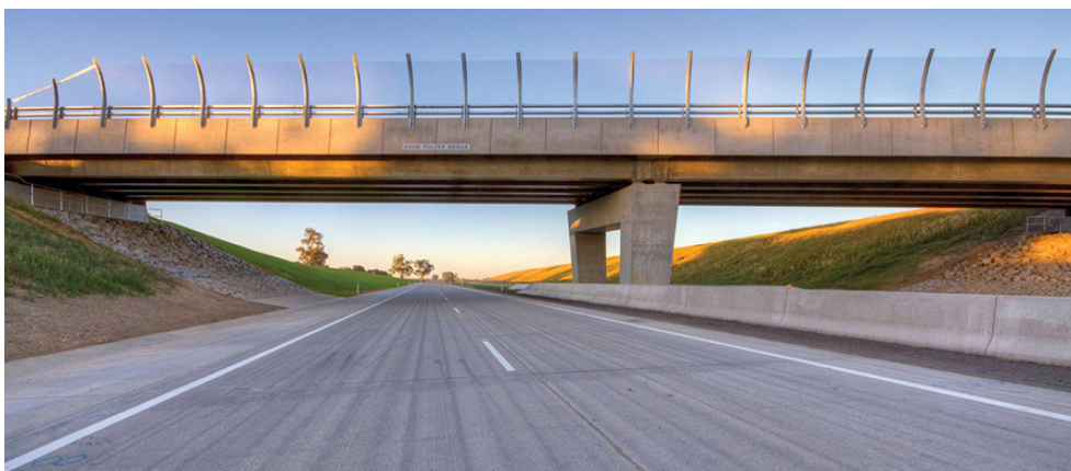
Figure 24: This bridge designed for the Hume Highway Duplication provides an example of visually transparent wire mesh throw screens, as well as of how the sense of openness under the bridge can be increased through the use spill-through abutments that avoid a 'tunnel feel'. It further illustrates an example of a simple and bold pier design (source: http://www.rms.nsw.gov.au/projects/planning-principles/centre-for-urban-design/achievements/images/hume-highway-duplication-2.jpg )
