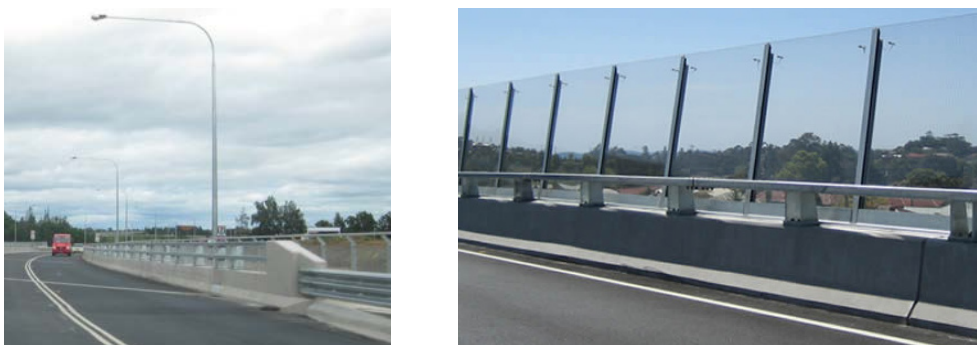
Figure 23: Examples of neat and simple integrated safety barriers between the carriageway and the shared path. Transparent throw screens provide for views into surrounding areas (source: http://www.noise-barriers.org/img/clear-sound-barrier.jpg )
