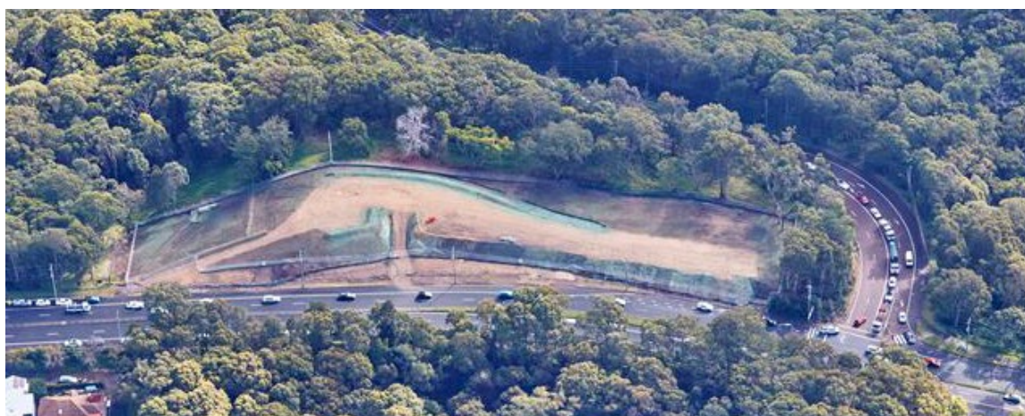
Figure 1.2 - House demolition site after completion of the works (taken 22 June 2021)
