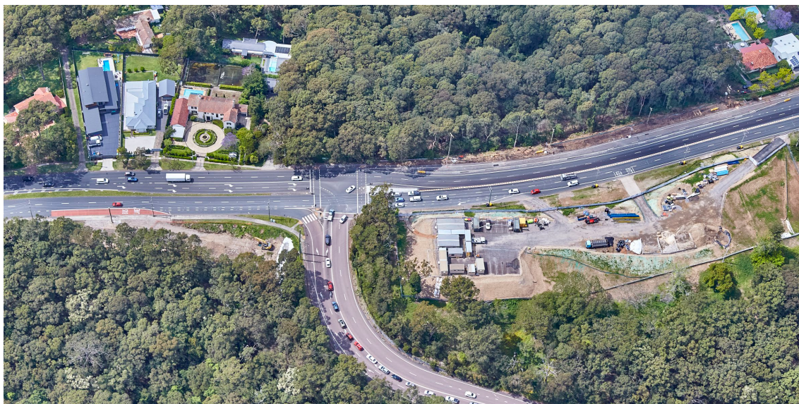
Figure 1.3 Southern Interchange utilities relocation works and site compound (taken 24 October 2021)
