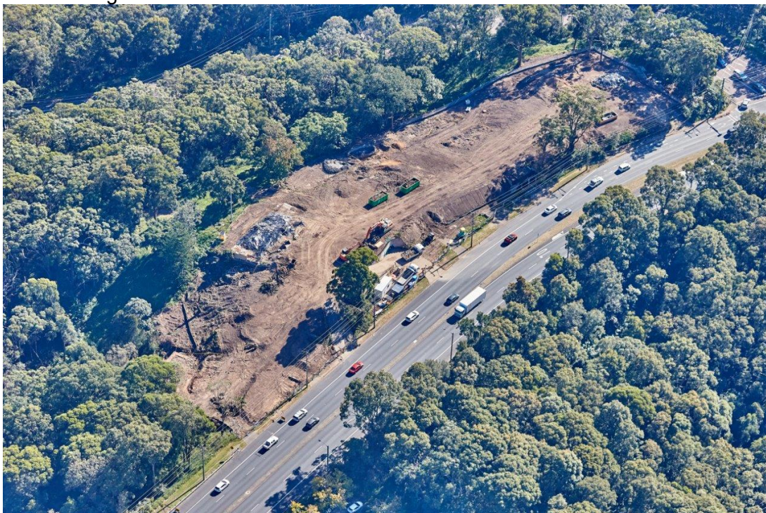
Figure 2 house demolition work
