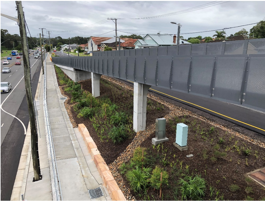
Photograph D.5 Drainage works and foot path under northern side of footbridge
