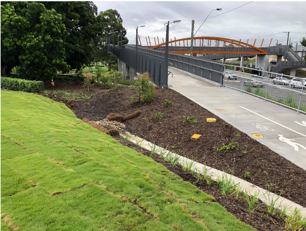
Photograph D.2 Completed revegetation around pedestrian Footbridge
