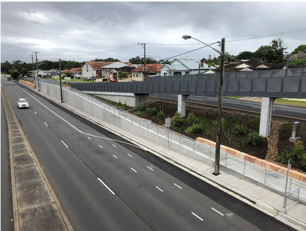
Photograph D.4 Completed footbridge (northern side)
