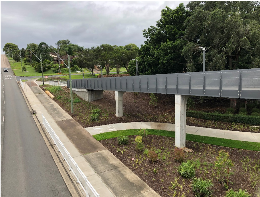
Photograph D.3 Completed revegetation around pedestrian footbridge
