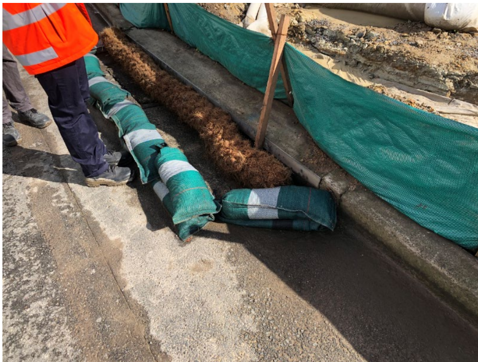
Photograph D.10 View of appropriate bunding and sedimentation controls implemented along Newcastle Road
