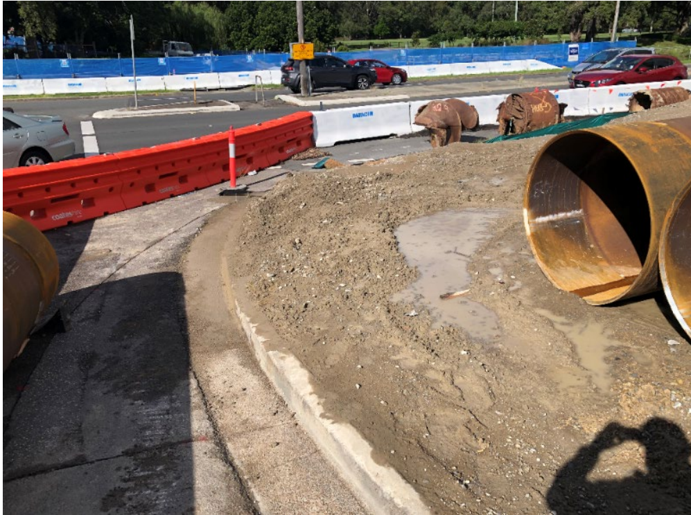
Photograph D.111 View of area where additional ESC required (Coles St / Newcastle Rd intersection)
