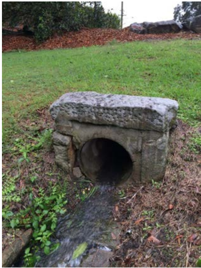
Plate 8 Sandstone and concrete drain
