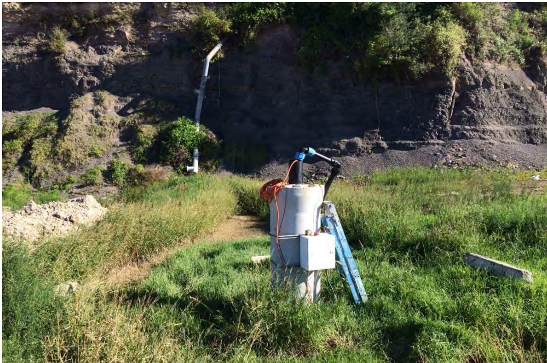
Plate 2 Intermediate leachate riser (EPL landfill premises area)
