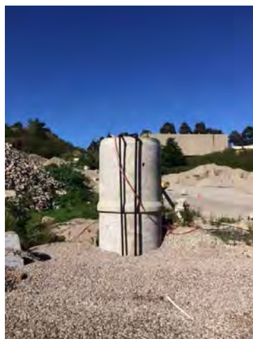
Plate 1 Main leachate extraction sump riser (facing south west)
